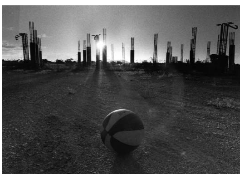
Construction of the "Dome" at Murray 1973
