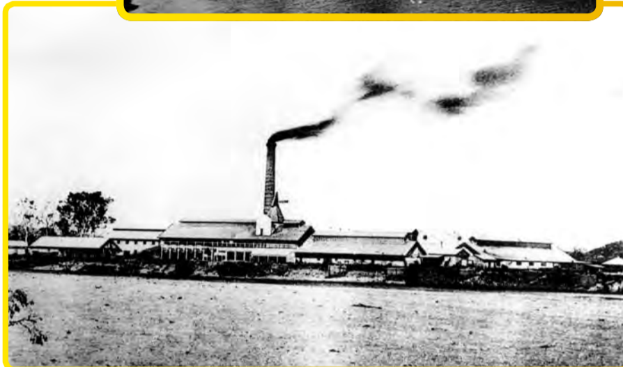
The historic 19th century meat works chimney will stay. IMAGE COURTESY OF CITYLIBRARIES' LOCAL HISTORY COLLECTION.
