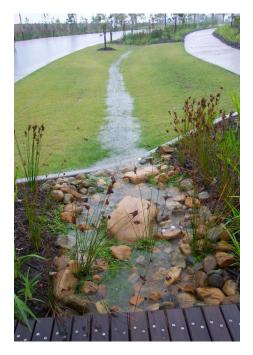
settling of sediments through the reduction of flow velocities and temporary detention. They can take various forms and can be used as permanent systems integrated into an urban design, or temporary measures to control sediment discharge during construction.
