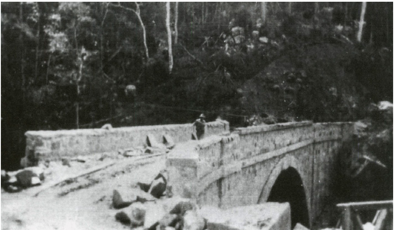
ca 1933 Little Crystal Creek, Mt Spec Road. The masonry arch bridges nears completion.
