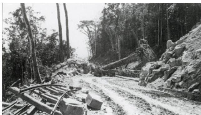
ca 1933 Mt Spec Road. View of a large maple balanced on the edge of Mt Spec Road during construction. Note the use of mining technology - tramlines and trolleys. Unknown, Thuringowa Collection
