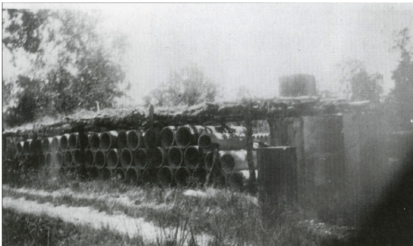
1932 Ollera Creek Pipeworks, Mt Spec Road. Pipeworks curing shed with stored pipes. Note the bough shelter over the curing concrete pipes. If the concrete dried too quickly, its strength was effected.
