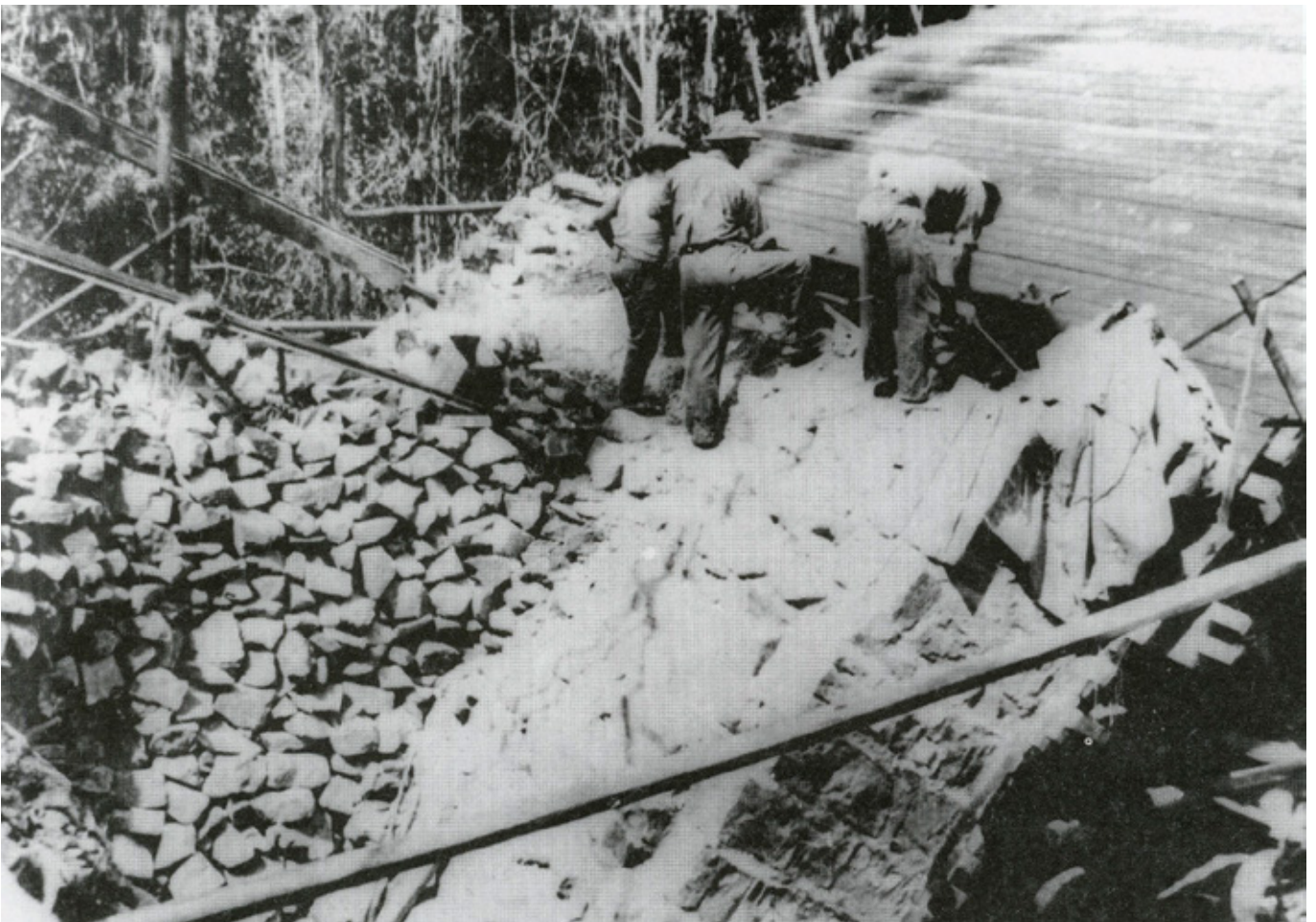
10 October 1932 Little Crystal Creek, Mt Spec Road. Abutment 'B' looking due south. Note the lagging put down on the formwork to haul the concrete when it was poured over the rock fill.
