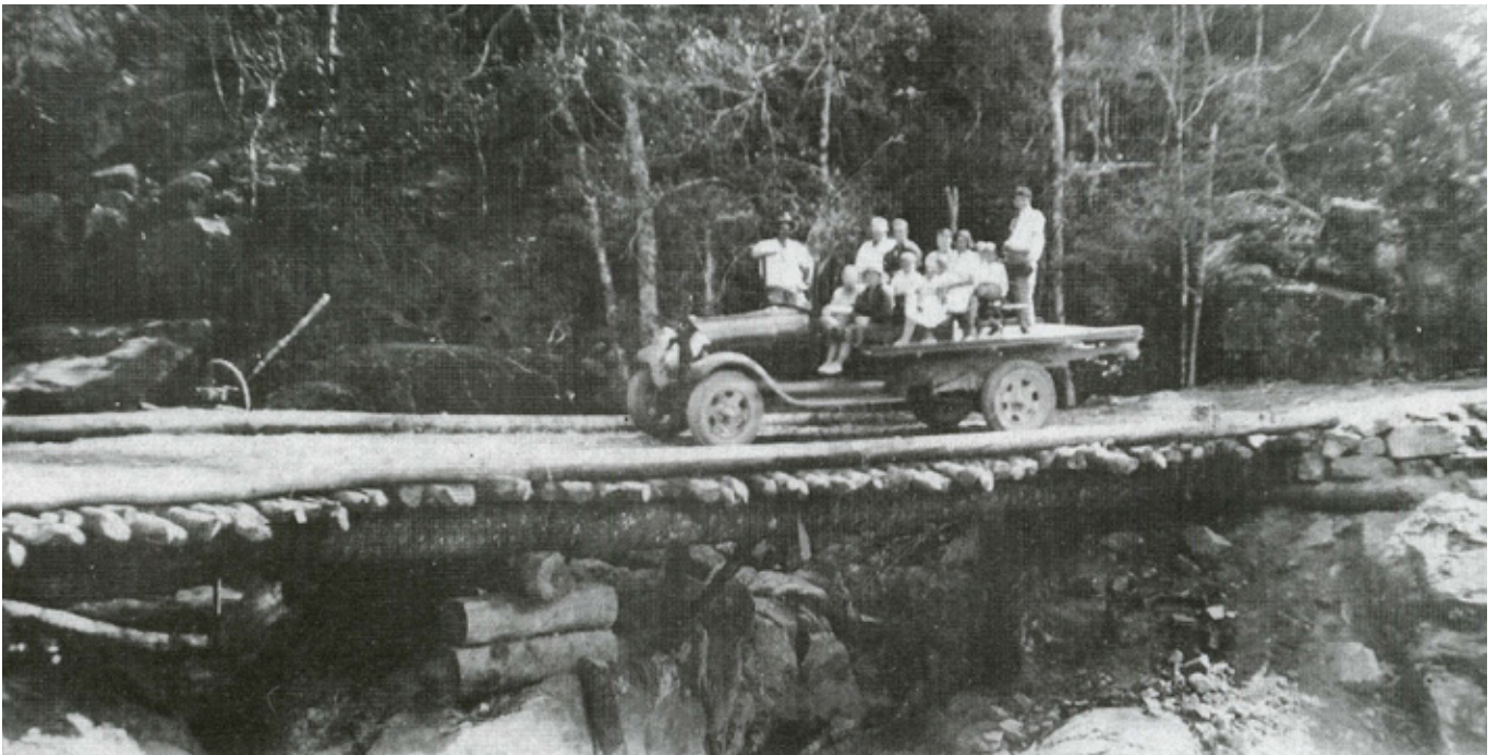
ca 1933 Little Saltwater (Crystal) Creek, Mt Spec Road. Ford truck on temporary bridge over Crystal Creek. This timber bridge was created to provide access to works beyond Little Crystal Creek while masonry arch bridge was still under construction.
