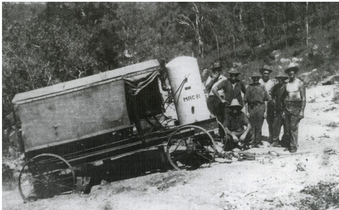
1931-35 Mt Spec Road. Main Roads Commission work cart with petrol powered compressor bogged in sand.
