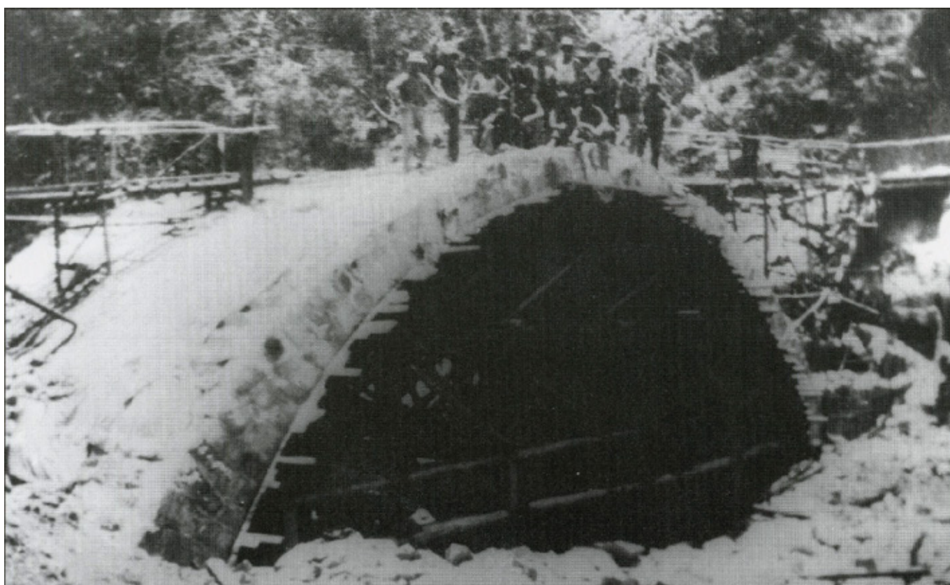
1932 Little Crystal Creek, Mt Spec Road. The masonry arch takes shape.
