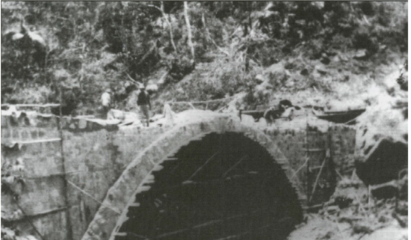
1933 Little Crystal Creek, Mt Spec Road. Both abutments almost complete.
