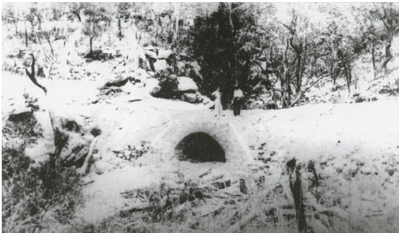
ca 1932 Mt Spec Road. A smaller masonry arch culvert at 17, 100 feet through chainage. Through chainage was measured from the beginning of the project at Moongabulla (near today's turnoff at Ollera Creek). There are several stone culverts like this. This particular one is at the base of the range. This was Job Number 117-501-4.
