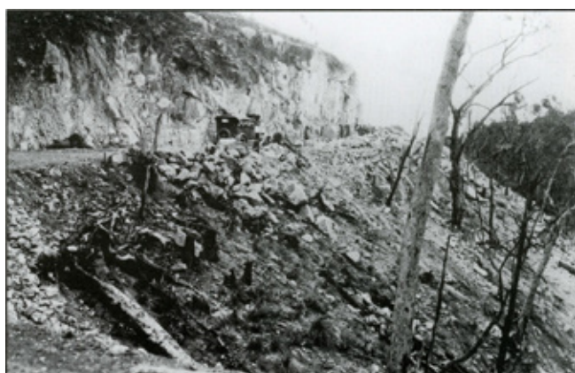
ca 1933 Mt Spec Road at 45,000 feet through chainage. Stone cutting during construction. Mrs McClelland noted that it was their car. McClelland, Thuringowa Collection
