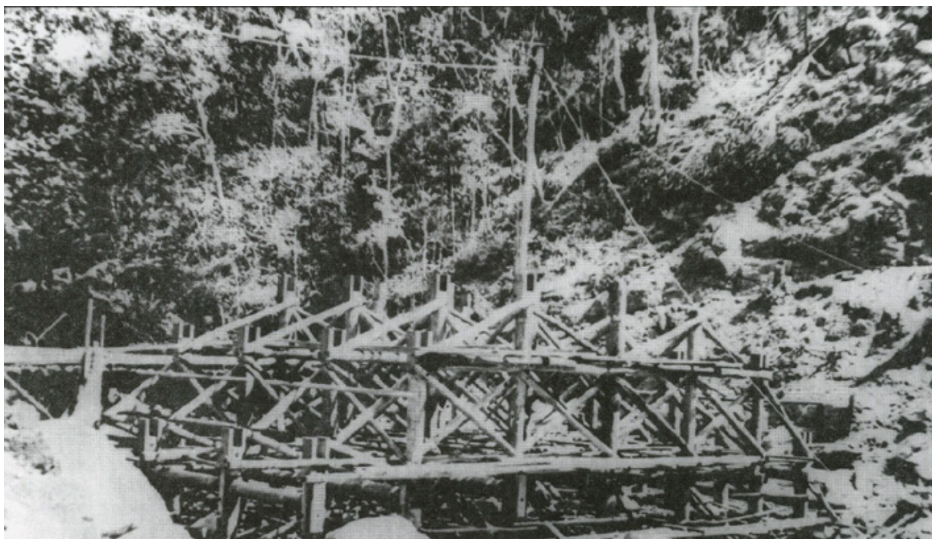
Early 1932 Little Crystal Creek, Mt Spec Road. Note the use of the round timbers for the initial framework of the masonry arch bridge.
