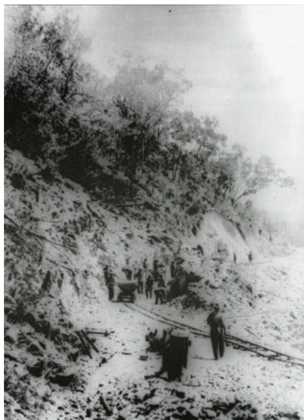
ca 1932 Mt Spec Road. Rock cutting between 20,000 feet and 20,200 feet through chainage.
