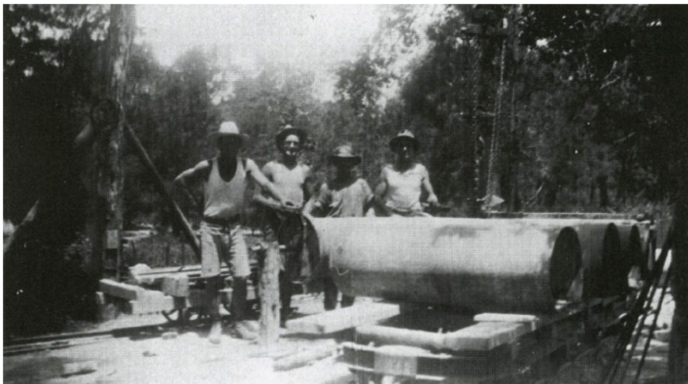
1932 Ollera Creek Pipe Works, Mt Spec Road. Ganger Albert Kerr was in charge of casting the hundreds of concrete pipes that carry water under the Mt Spec Road. The photograph shows the assembling of the inner and outer moulds.
