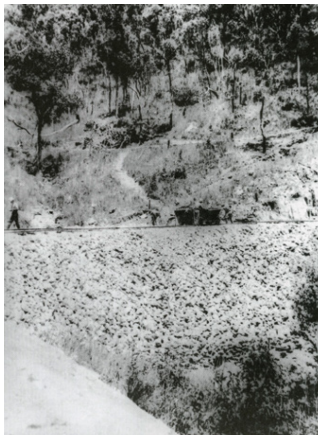
ca 1932 Mt Spec Road. Rock fill through chainage approximately 19,900 feet. Note the use of tramlines and trolleys and rope to mark the line of construction.
