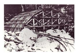
Rock was then filled behind the arch and lagging put down to hold the concrete when it was poured. Once the arch was in place the abutments were completed and the road was laid. Perhaps it is the appearance of the bridge that calls to mind earlier stone bridges built by convicts in the southern parts of Australia.
