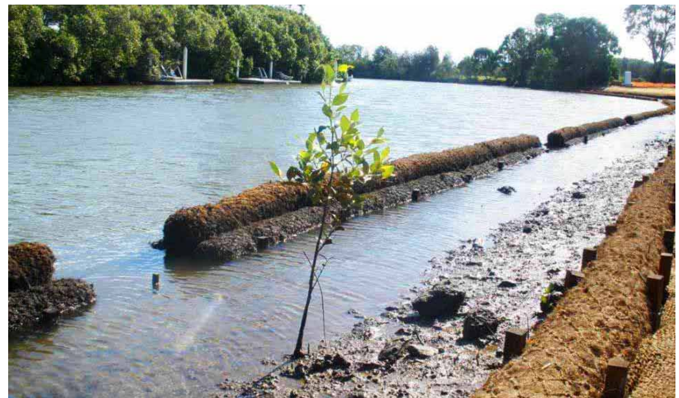
Figure 46: Soft erosion structure (Gold Coast) positioned in front of mangrove zone to prevent erosion and bank under slump. Structure is made from a natural fibrous husk, designed to be pegged in place for aquatic vegetation behind structure to take hold. This product will break down over time. Photo source – N. Waltham
