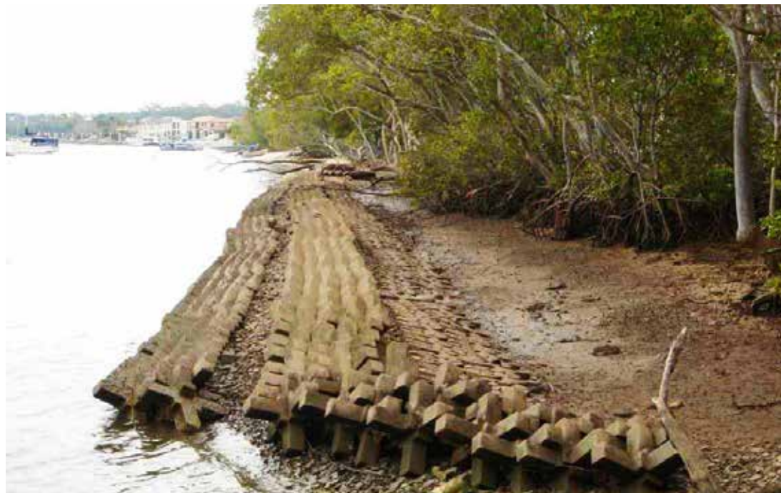
Figure 43: Concrete erosion structure (Gold Coast) positioned in front of mangrove zone to prevent erosion and bank under slump. This structure (A-Jacks) is designed to be interlocking, increasing structural integrity of the wall. These structures provide a high level of complexity for aquatic organisms to exist, mostly intertidal snails, bivalves and encrusting algae. Photo source – N. Waltham
