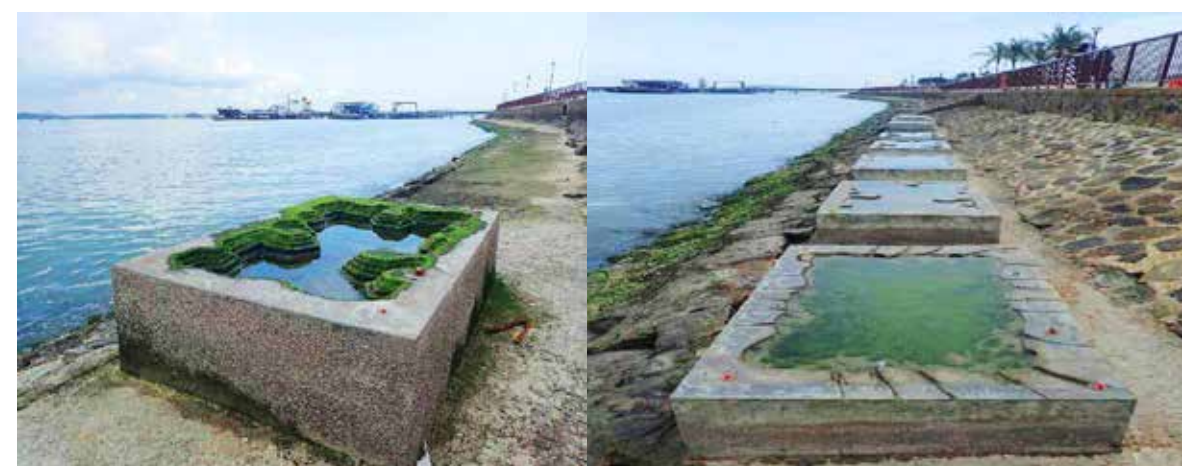
Figure 48: Concrete seawalls with installed in Singapore to create artificial intertidal rock pool habitat to increase opportunities for aquatic organisms. Photo source – N. Waltham
