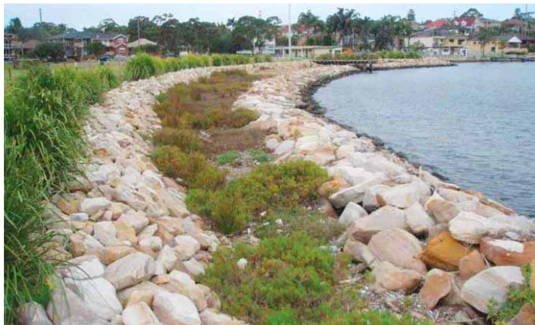
Figure 44: Example of living shoreline constructed at Kogarah Bay, Georges River, showing the benching seawall design supporting saltmarsh vegetation (Office of the Environment and Heritage, 2012, p. 35)
