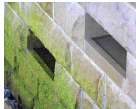
Figure 47: Example of constructed voids (here with pools that form in the base of the block void, in block seawall in Sydney harbor (Office of the Environment and Heritage, 2012)
