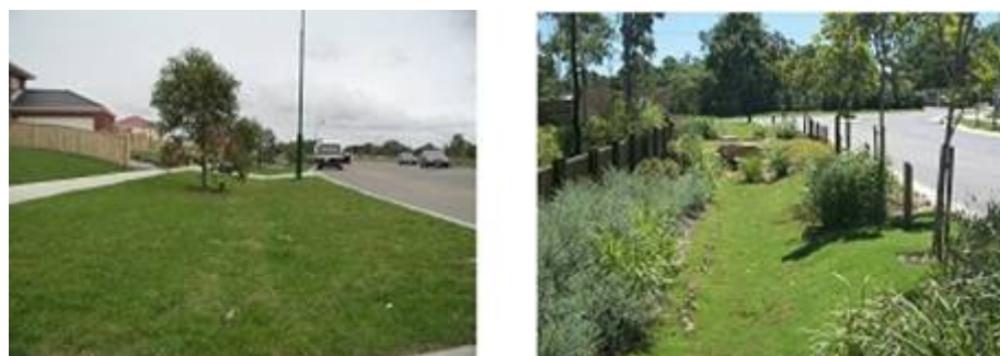
Plate 2-4: Typical sections for Swale 1 (left) and Swale 2 (right) (Note that Swale 1 also requires provision for traffic control and Swale 2 requires provision for pedestrians)
