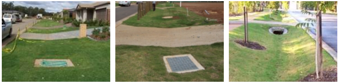
Plate 2-2: At-grade (left) under construction with trees yet to be established, pre-constructed 'at-grade' (centre) and elevated driveway crossings to allow vehicle access across swales
