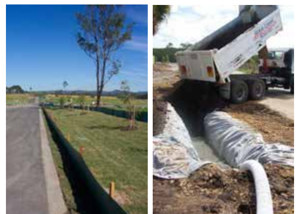
Plate 3-5: Bioretention Swale Functional Installation
