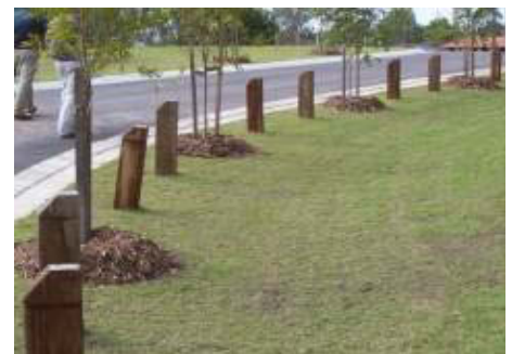
Plate 2-5: Traffic bollards mixed with street trees to protect swale from vehicles
