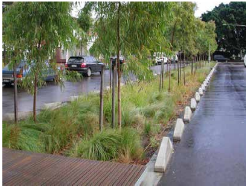
Plate 3-3: Median Strip Bioretention applications
