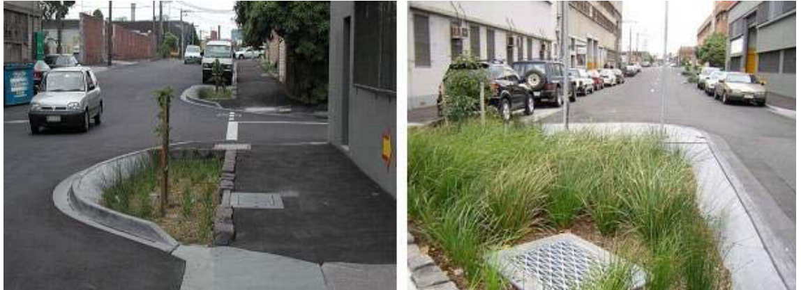
■ Plate 5-6: Retrofitted Bioretention System in a Street
