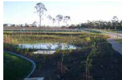
Plate 6-10: Constructed Wetland Functional Installation
