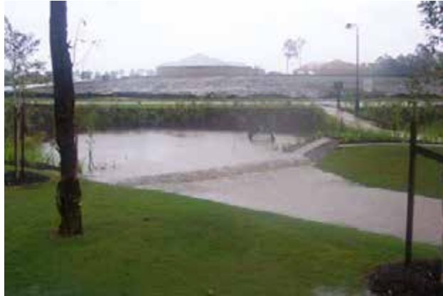
Plate 6-2 Inlet zone bypassing major design flows around wetland.
