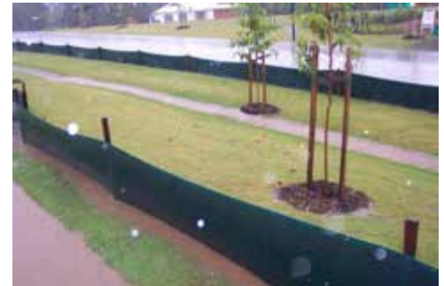
Plate 3-6: Bioretention Swale Sediment & Erosion Control
