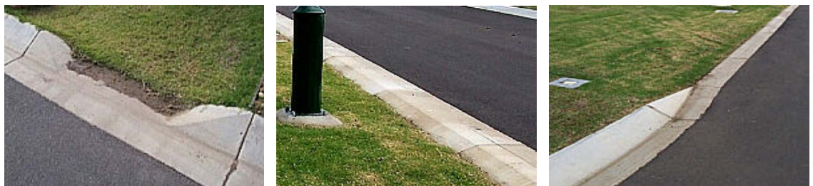
Plate 2-3: Kerb arrangements to promote distributed flow into swales
