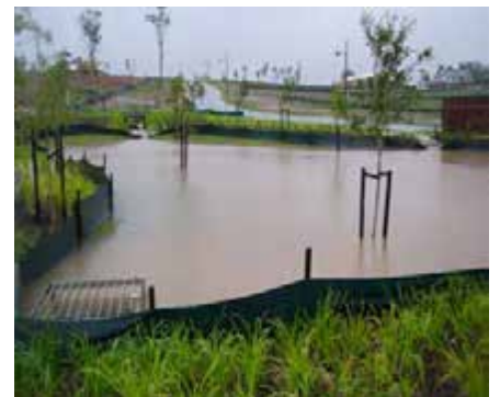
■ Plate 5-5 : Bioretention Basin Sediment & Erosion Control
