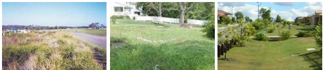
Plate 2-1: Swale systems: heavily vegetated (left), use of check dams (centre), grass swale with elevated crossings (right)
