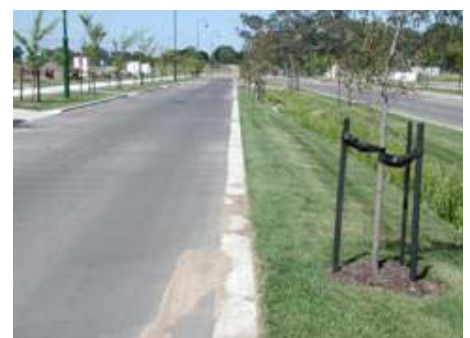
Plate 3-2: Flush Kerb without Setdown, showing Sediment Accumulation on Road
