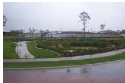
Plate 6-10: Constructed Wetland Sediment & Erosion Control Operation
