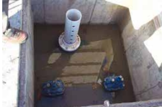
Plate 6-6: Macrophyte Zone Outlet Arrangement
