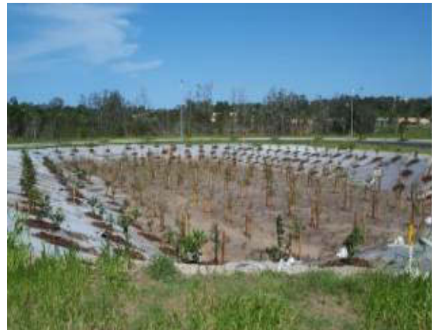
■ Plate 5-6: Plant Establishment Period in Bioretention
