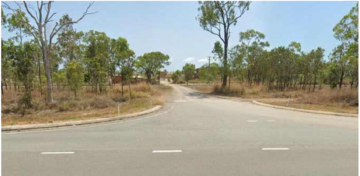
Figure 6. Bruce Highway looking at site access
