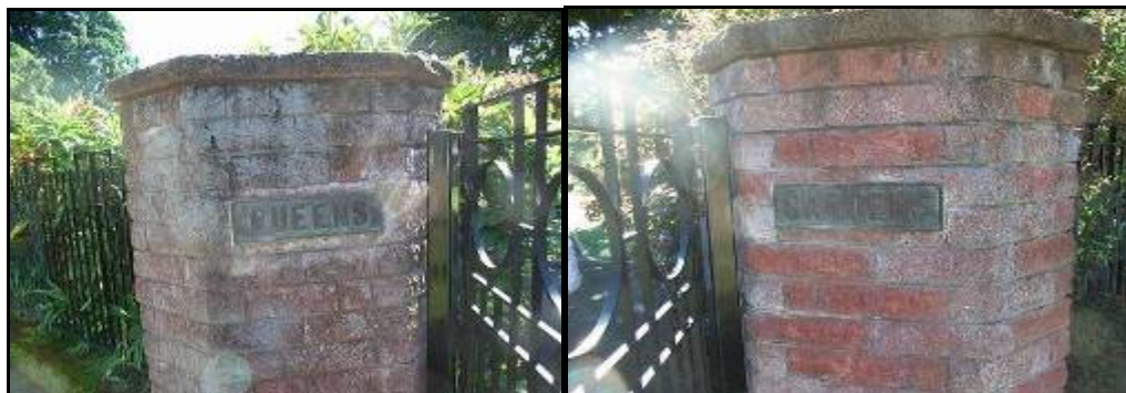
Figure 3.33 Detail of plaques mounted either side of Paxton Street Entrance (ERM 2010)
