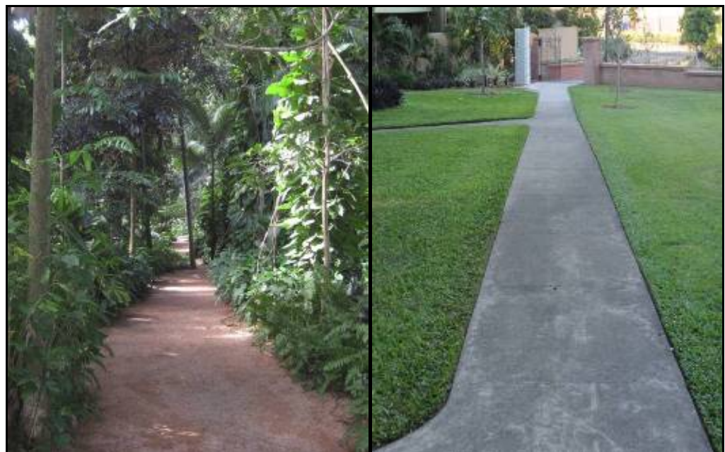
Figure 3.42 Pathways: Red “Cracker Dust” (left) and concrete (right)
