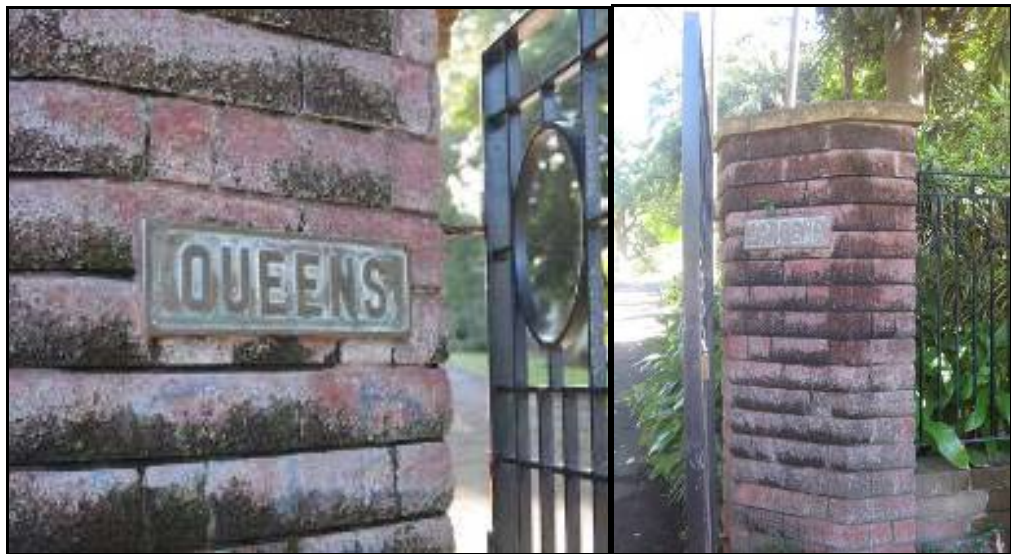
Figure 3.35 Entrance plaques and piers (ERM 2010)
