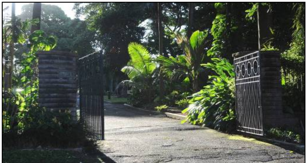
Figure 3.32 Paxton Street Entrance, featuring double hung powder coated steel gates attached to concrete brick piers (ERM 2010).
