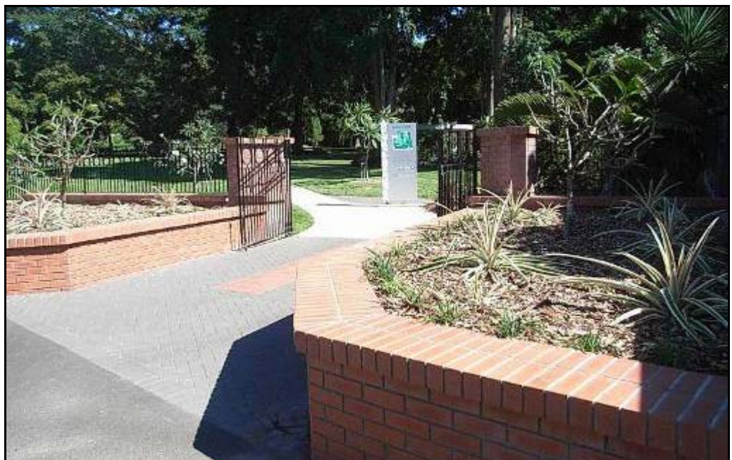
Figure 3.37 New Gregory Street entrance is similar in intent to the original design, although constructed in clay brick (ERM 2010)
