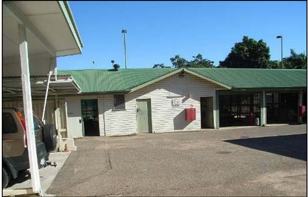
Figure 3.24 Workshops viewed from south. (ERM 2010)
