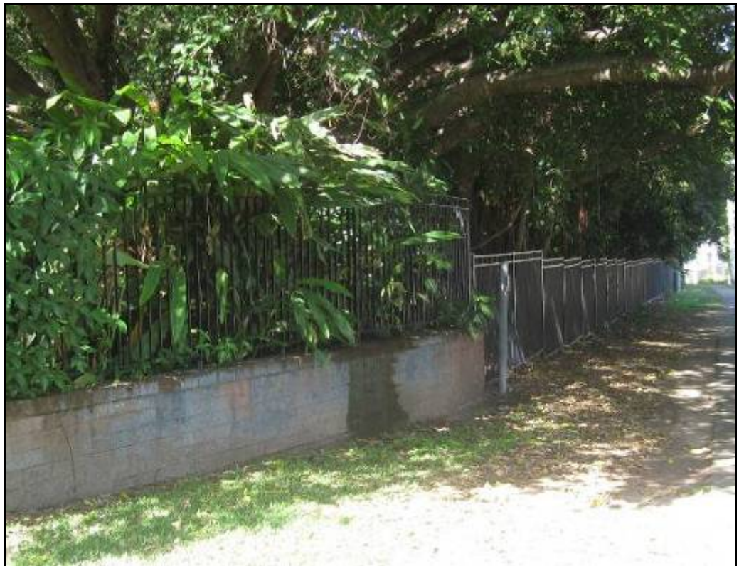
Figure 3.38 Fencing on Paxton Street
