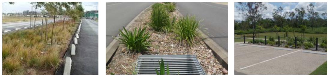
Plate 3-1: Kerb Arrangements with Breaks and Flush Kerbs to Distribute Inflows on to Bioretention Swales and Prevent Vehicle Access
