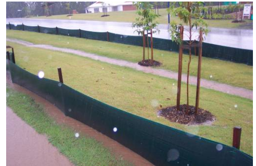
Plate 3-6: Bioretention Swale Sediment & Erosion Control
