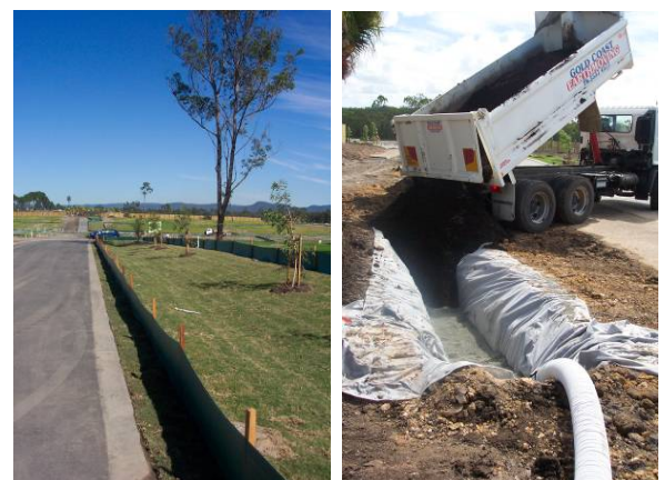
Plate 3-5: Bioretention Swale Functional Installation
