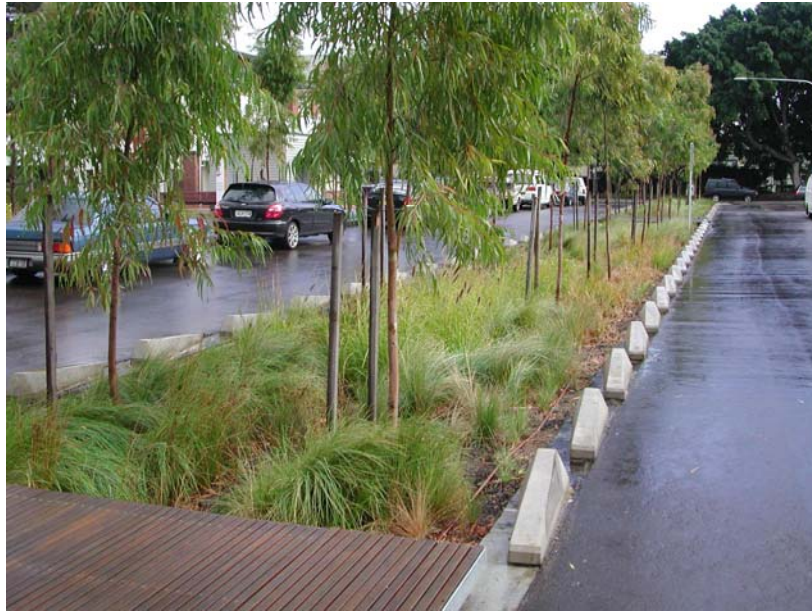
Plate 3-3: Median Strip Bioretention applications
