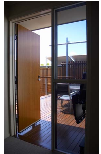
Use of louvres instead of fixed glass would enhance cross-ventilation
