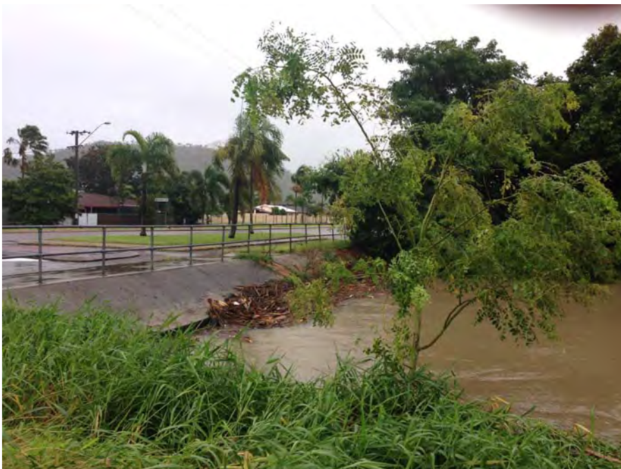
Photo 2 – Bayswater Road Crossing at 09.56 AM on 13 th Apr 2014.
