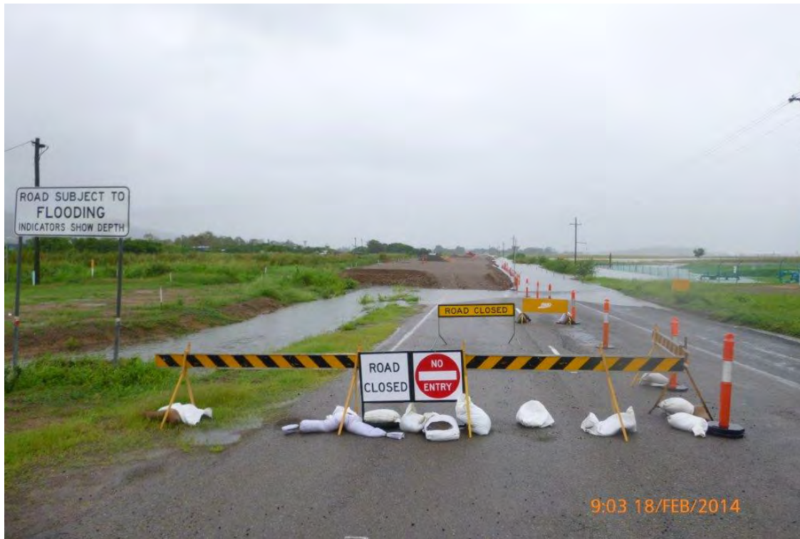
Photo 1 – Approach to Blakeys Crossing at 09.03 AM on 18 th Feb 2014.
