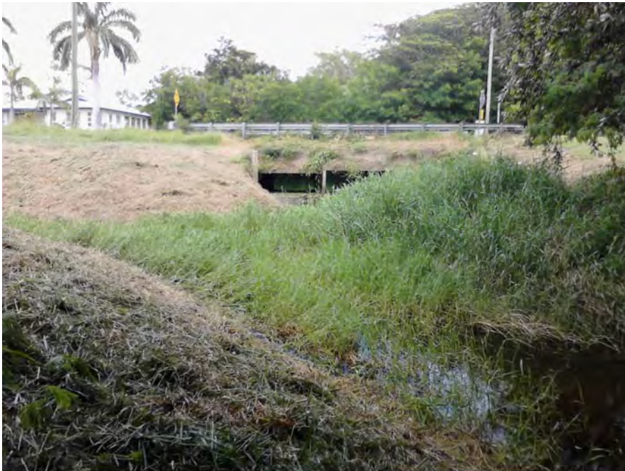
Photo 8 – Louisa Creek channel confluence at Banfield Drive / Dalrymple Road (looking towards Banfield Drive)
