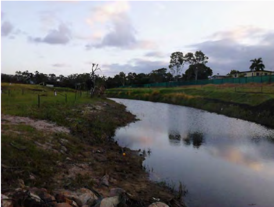
Photo 13 – Louisa Creek Diversion looking upstream
