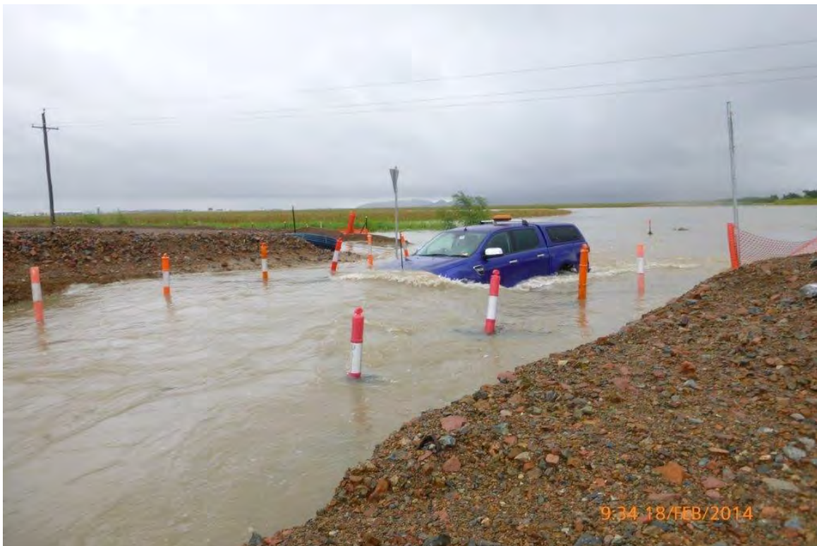
Photo 6 – Blakey St at Blakeys Crossing at 09.34 AM on 18 th Feb 2014.
