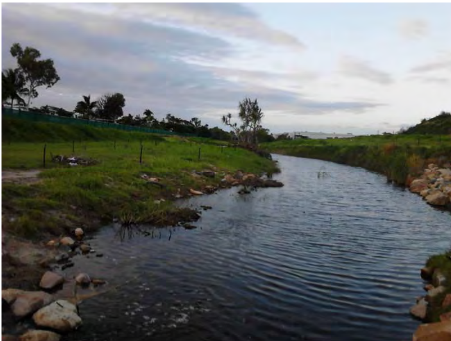
Photo 14 – Louisa Creek Diversion looking downstream
