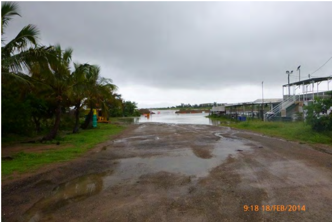
Photo 5 – Blakey St at Blakeys Crossing at 09.18 AM on 18 th Feb 2014.
