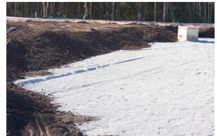
■ Plate 5-4: Bioretention Basin Functional Installation
