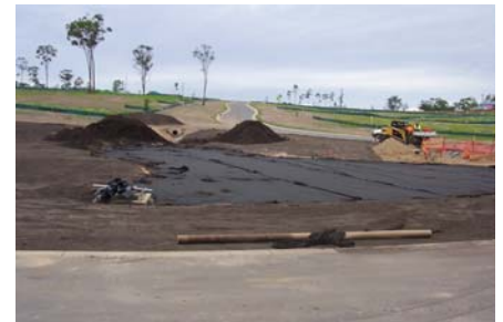
■ Plate 5-4: Bioretention Basin Functional Installation
