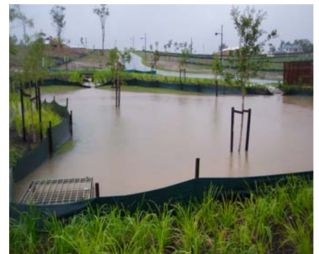
■ Plate 5-5 : Bioretention Basin Sediment & Erosion Control
