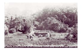
All that changed when relief workers built the road. The work was hard and living conditions were difficult and isolated. Few mechanical aids were used and workers cleared the rainforest with picks and shovels. Explosives were used to blast areas of rock and horse drawn scoops, wheelbarrows or mining trolleys on small pieces of portable track removed the rock. The gravelled road was officially opened on 18 July 1937.
