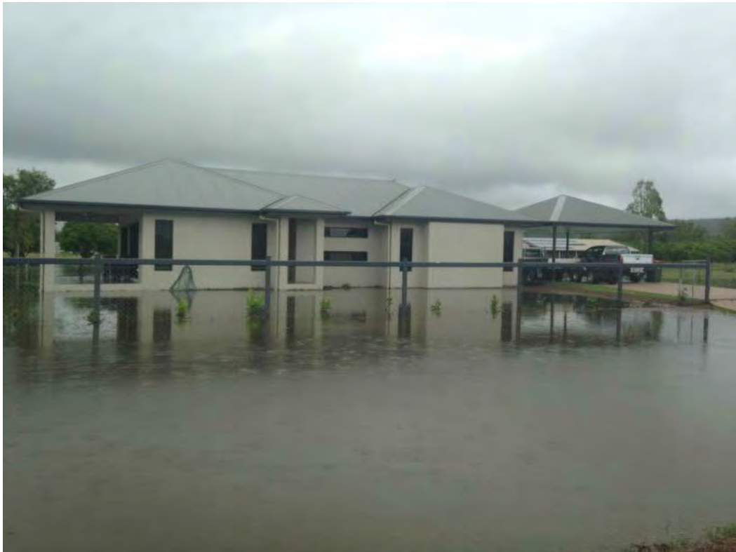
PIC 13: From Corser Drive looking towards Lot 30 about 2hrs after rain stopped.
