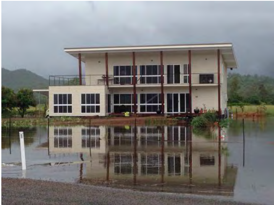
PIC 14: From Corser Drive looking towards Lot 28 about 2hrs after rain stopped.
