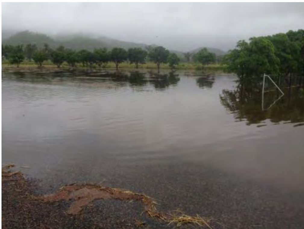
PIC 10: From Corser Drive looking towards Lot 27 about 2hrs after rain stopped.
