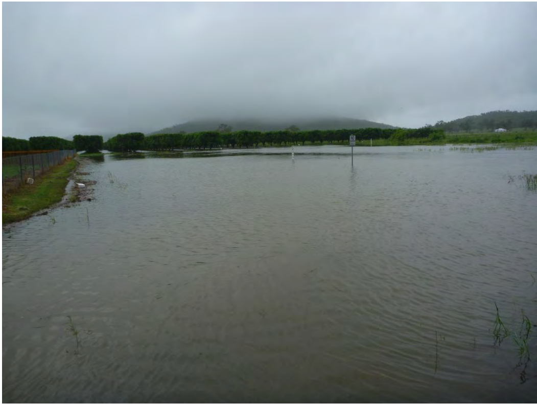
PIC 5: Lot 15 – Retention basin about 2hrs after rain stopped.
