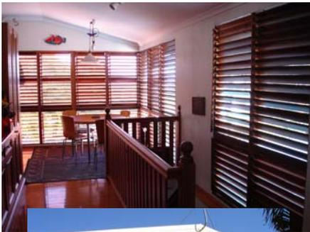
Adjustable, floor to ceiling timber louvres on two of the walls in the new extension not only enhance views, but improve cross ventilation and minimise heat gain.
