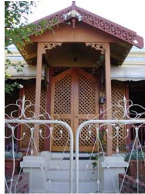
When closed, the lattice provides a privacy screen that allows the breeze to flow to the
