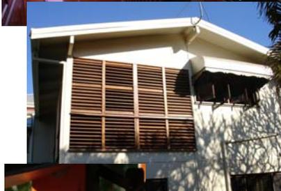
Solid louvres (in this case timber) block out low angle sun and heat from the east (morning) and west (afternoon).
