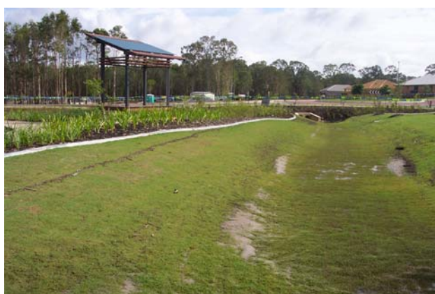
Plate 6-7: Turfed constructed wetland high flow bypass weir configuration.
