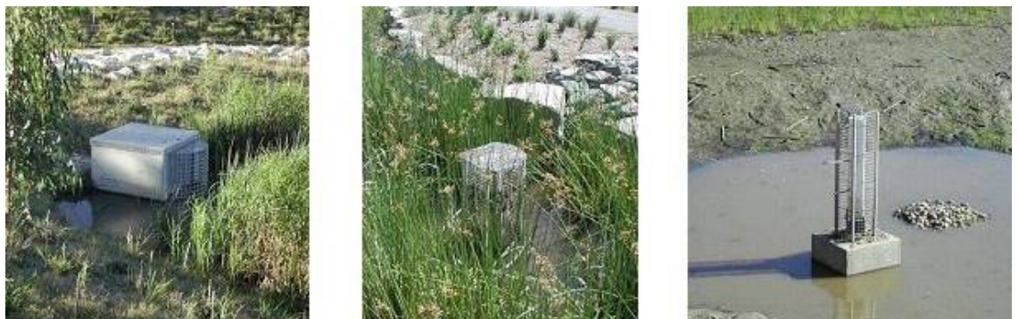
Plate 6-5: Example Outlet Riser Assemblies with Debris Guards
