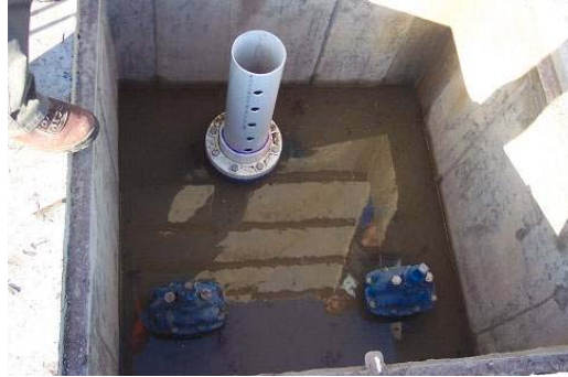
Plate 6-6: Macrophyte Zone Outlet Arrangement
