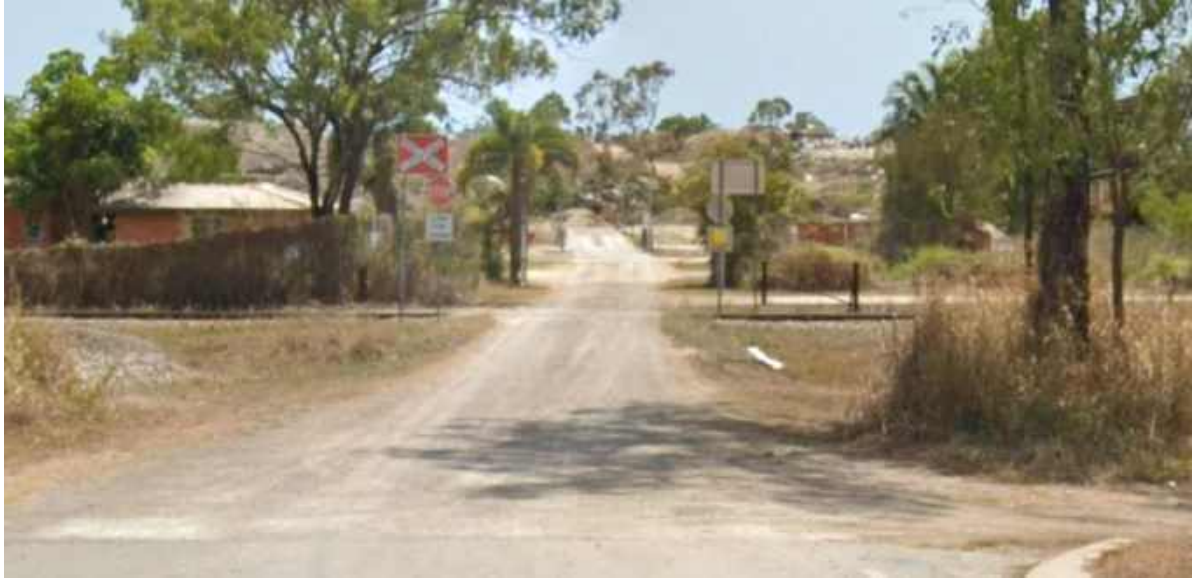
Figure 13. Existing Railway Crossing with stop sign control
