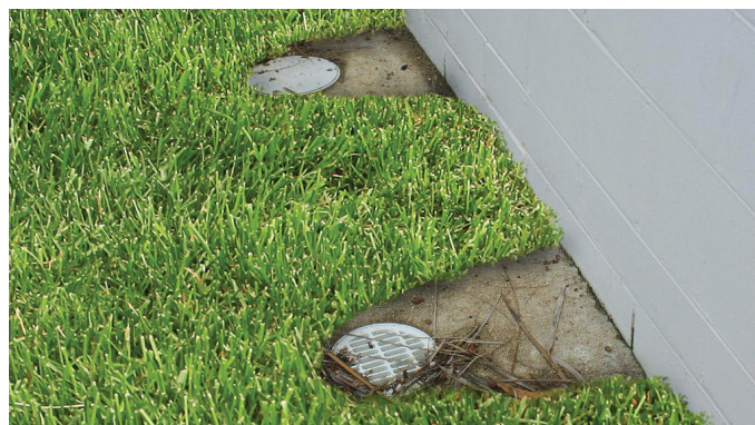
Landscaping that incorrectly directs stormwater into the ORG.
