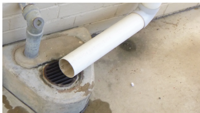
Illegal plumbing. The pipe from the right channels stormwater into the ORG.
