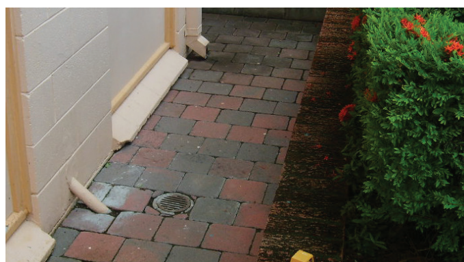
Paving that incorrectly channels water into the wastewater network.
