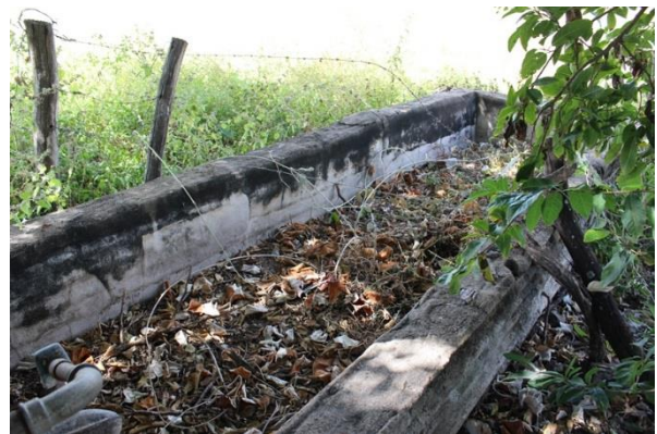
Figure 41: Water trough at the tanks.
