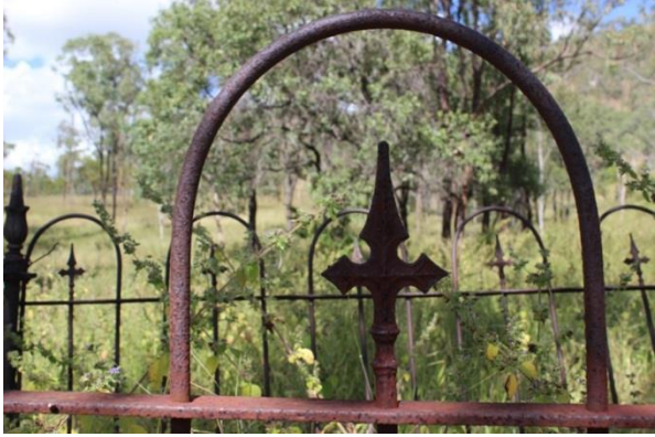
Figure 51: Detail of the fence surround.
