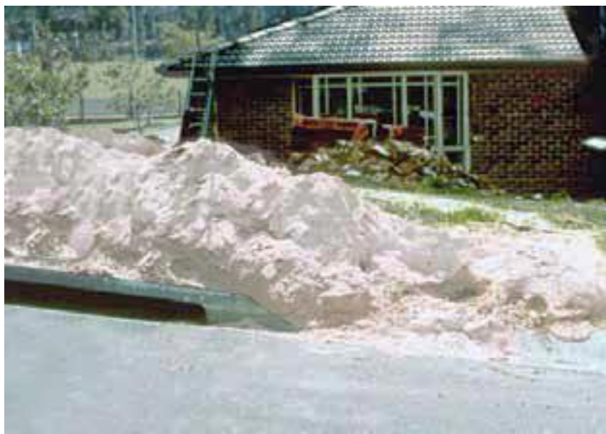
Poor stockpile control. Photo courtesy of Catchments and Creeks PTY Ltd
