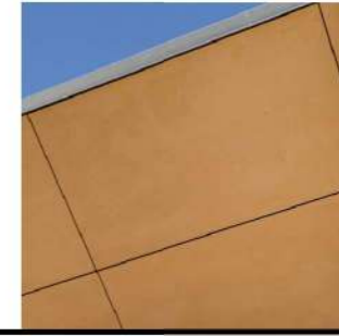
SFT-01 PRE-FINISHED FIBRE CEMENT SOFFIT
