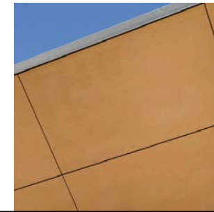
SFT-01 PRE-FINISHED FIBRE CEMENT SOFFIT
