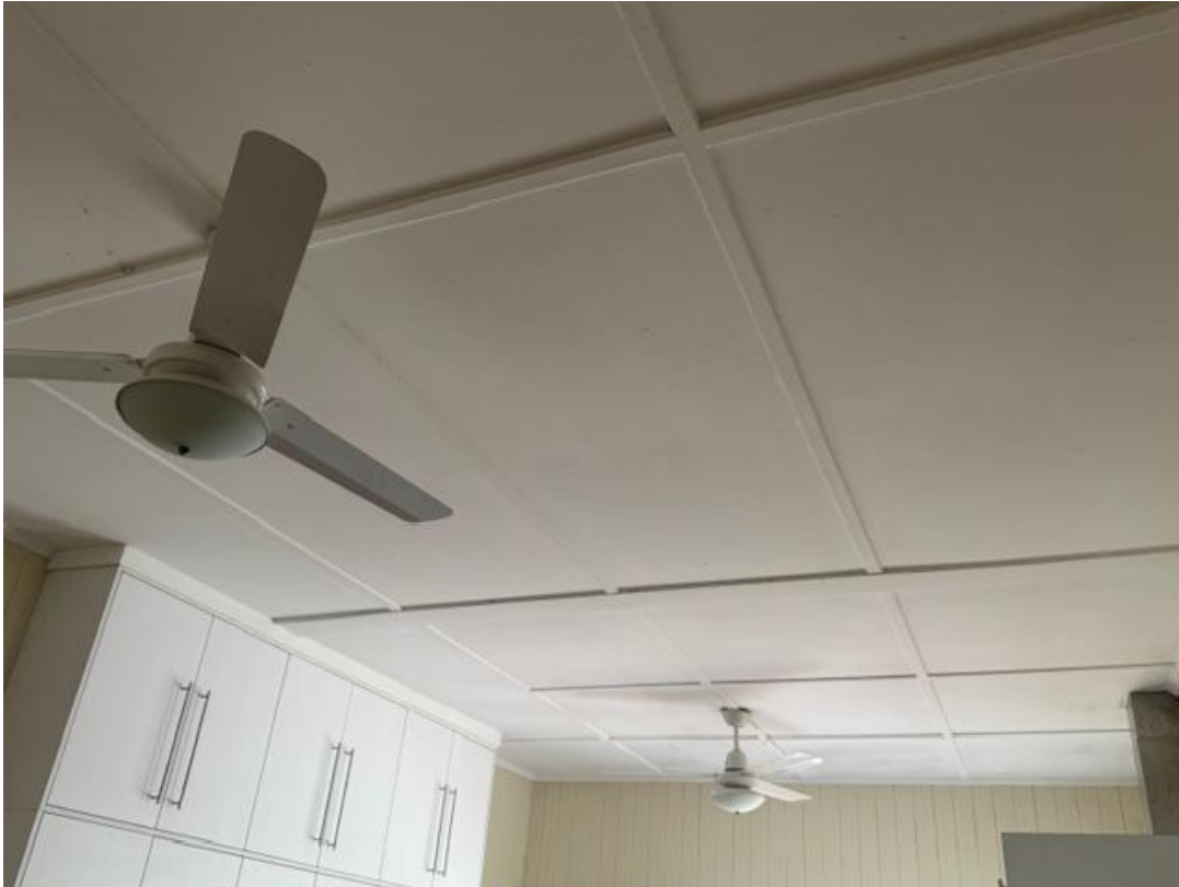
Figure 11 Internal Ceiling in Kitchen
