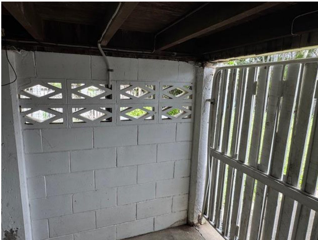
Figure 4 Un-reinforced 100mm screen blocks
