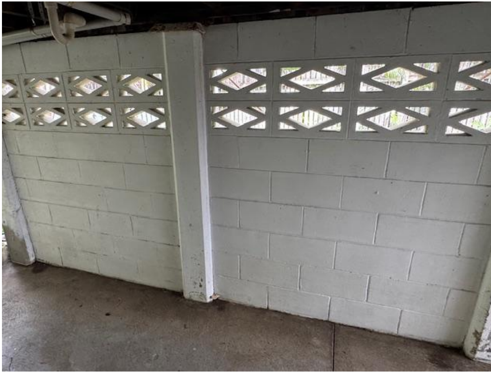
Figure 5 Un-reinforced 100mm screen blocks
