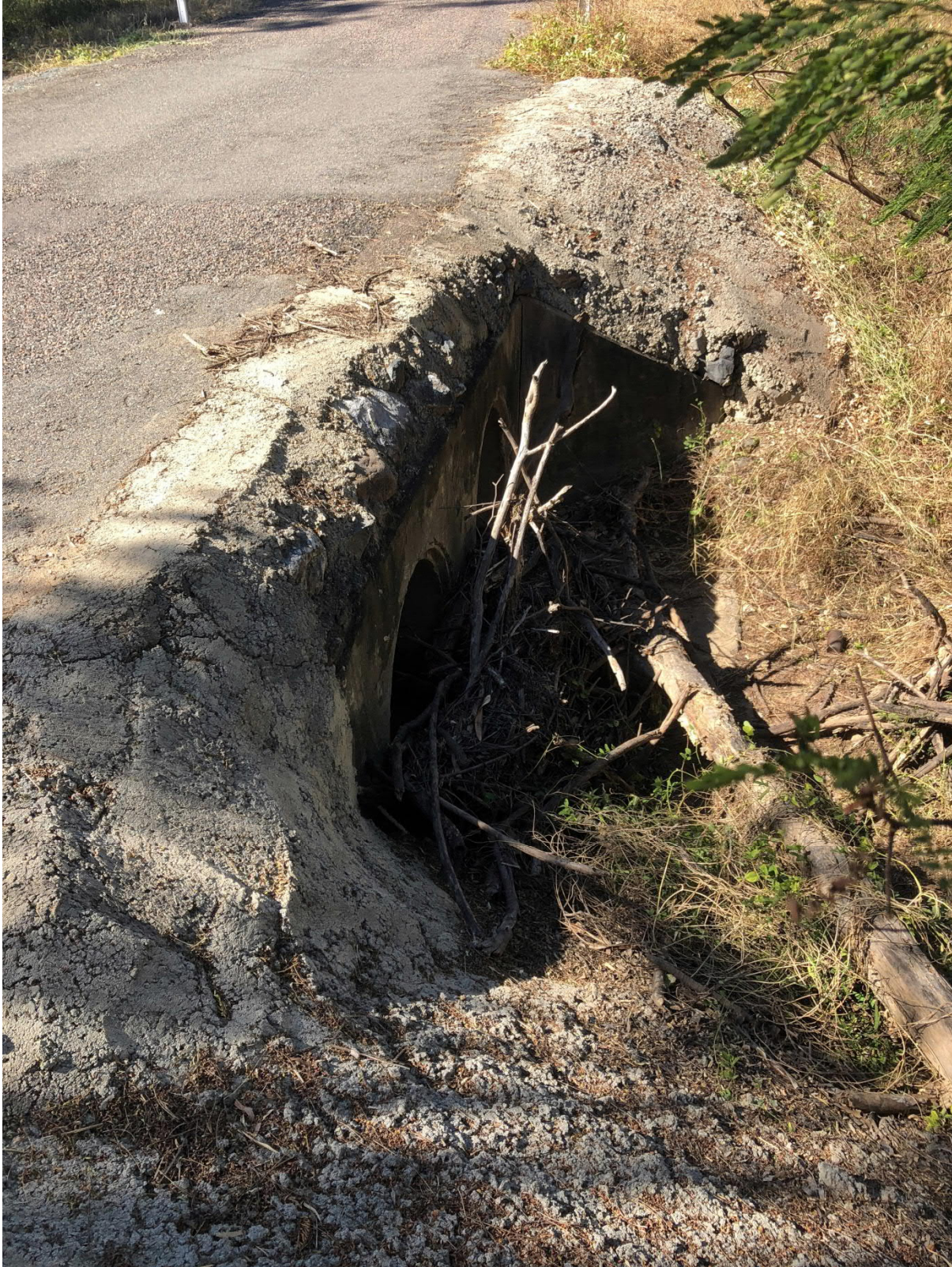
Photo 1 Sky Diver Road Culvert – 50% Blocked
