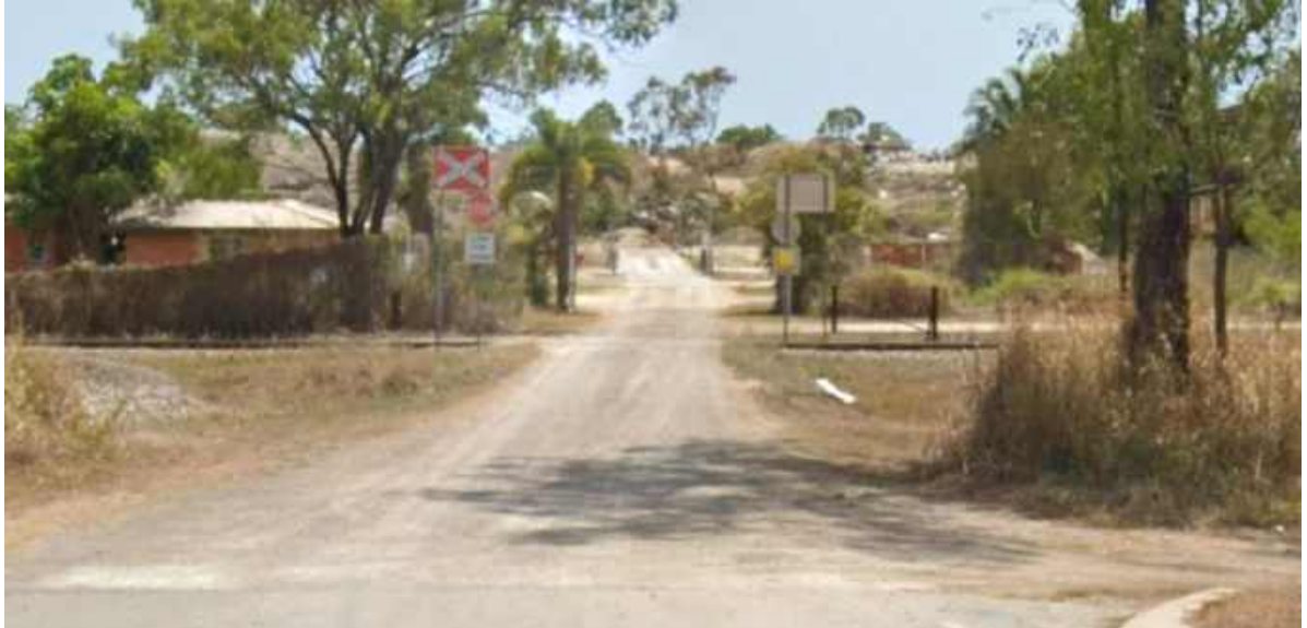
Figure 13. Existing Railway Crossing with stop sign control
