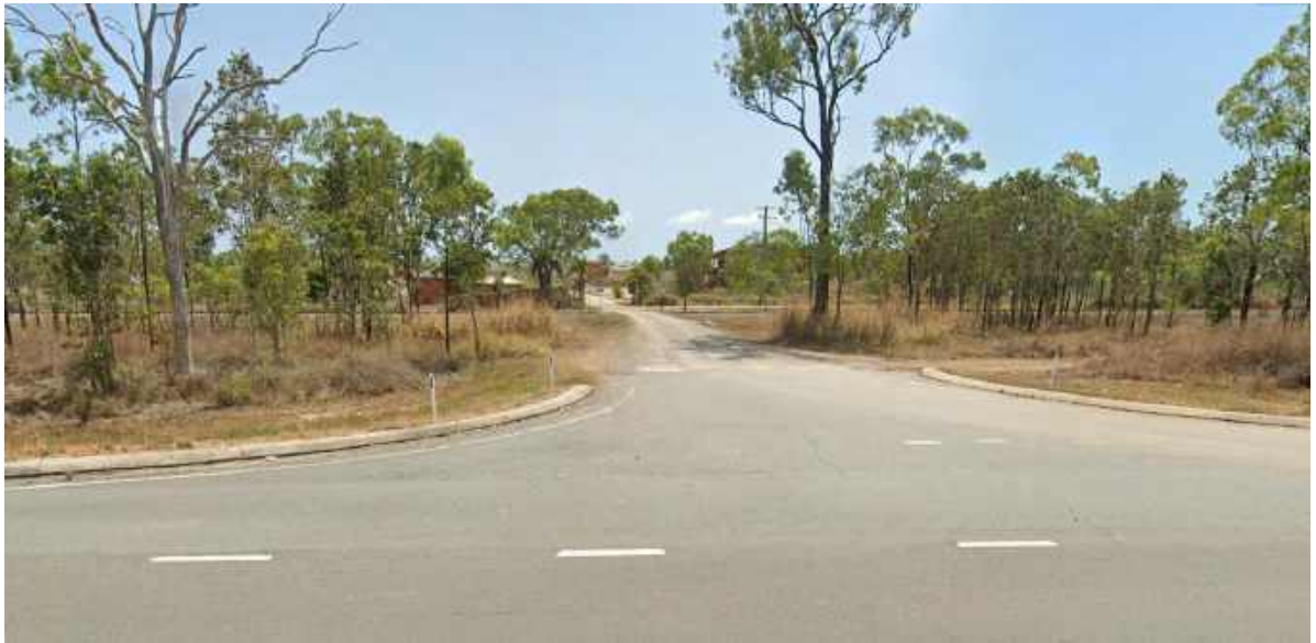
Figure 6. Bruce Highway looking at site access
