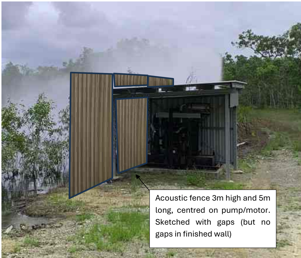
Figure 8: Acoustic Screen for Pump (Conceptual layout)
