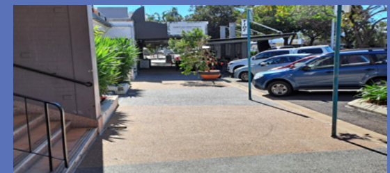
Mitchell, Gregory, and Eyre Street Pathway Upgrade.
