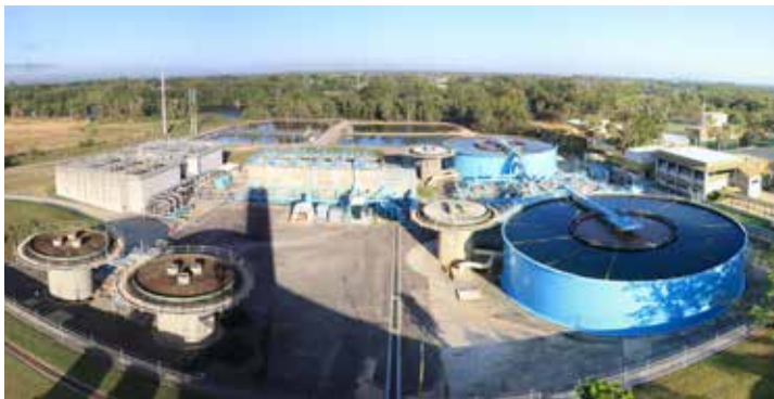
Douglas Water Treatment Plant
