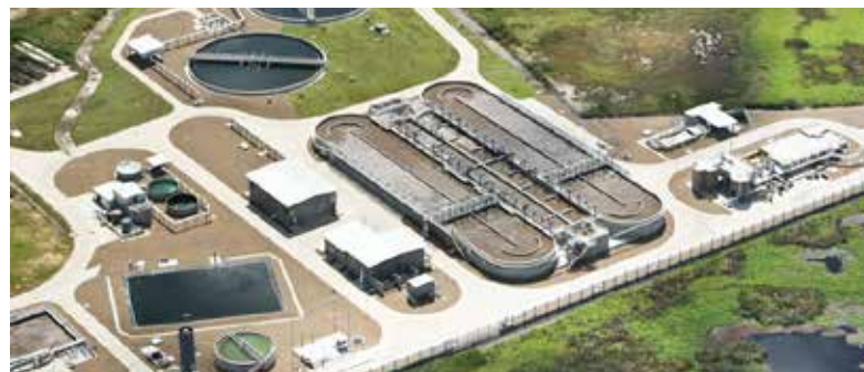
Mount St John Sewage treatment Plant
