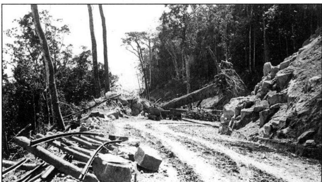
ca1933 Mt Spec Road. View of a large maple balanced on the edge of Mt Spec Road during construction. Note the use of mining technology – tramlines and trolleys.
