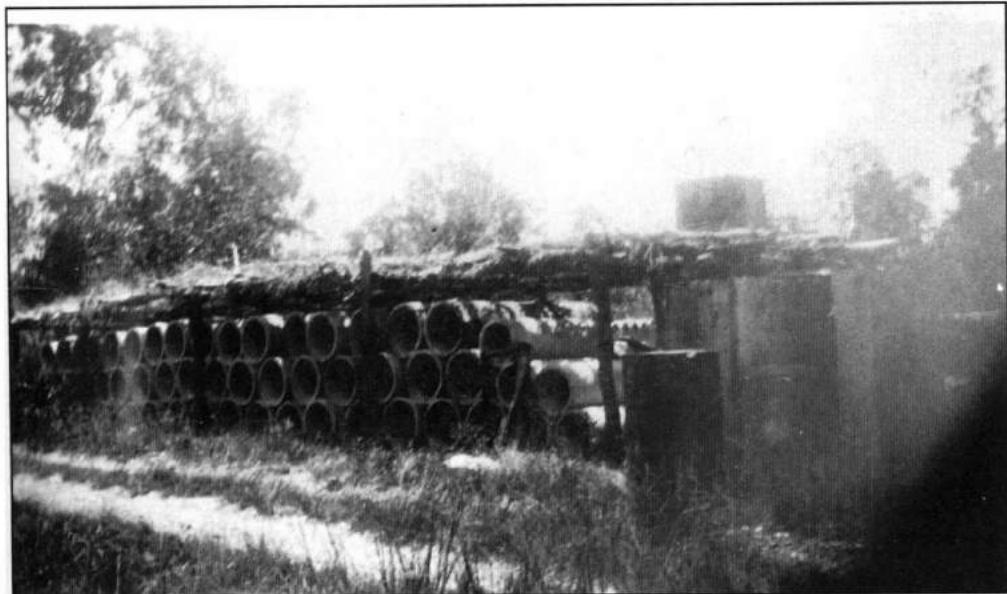
1932 Ollera Creek Pipeworks, Mt Spec Road. Pipeworks curing shed with stored pipes. Note the bough shelter over the curing concrete pipes. If the concrete dried too quickly, its strength was effected.
