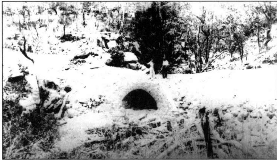
ca 1932 Mt Spec Road. A smaller masonry arch culvert at 17,100 feet through chainage was measured from the beginning of the project at Moongabulla (near today's turnoff at Ollera Creek). There are several stone culverts like this. This particular one is at the base of the range. This was Job Number 117-501-4.
