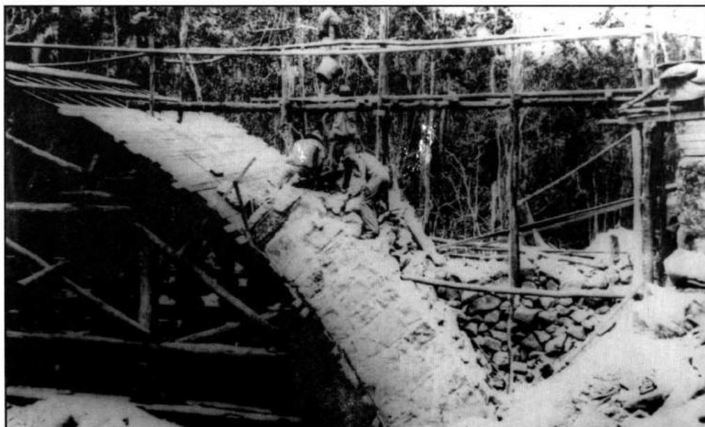
10 October 1932 Little Crystal Creek, Mt Spec Road. Abutment 'B' looking due South. Note the rock fill behind the arch.
