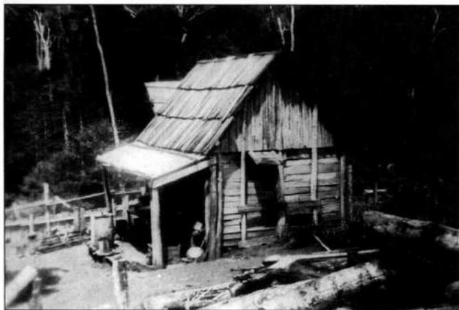
1911 Mt Spec. Jack Johnstone's Hut. The walls and roof are made of maple slabs. In the mid 1980s, the gravel foundations were still discernible.
