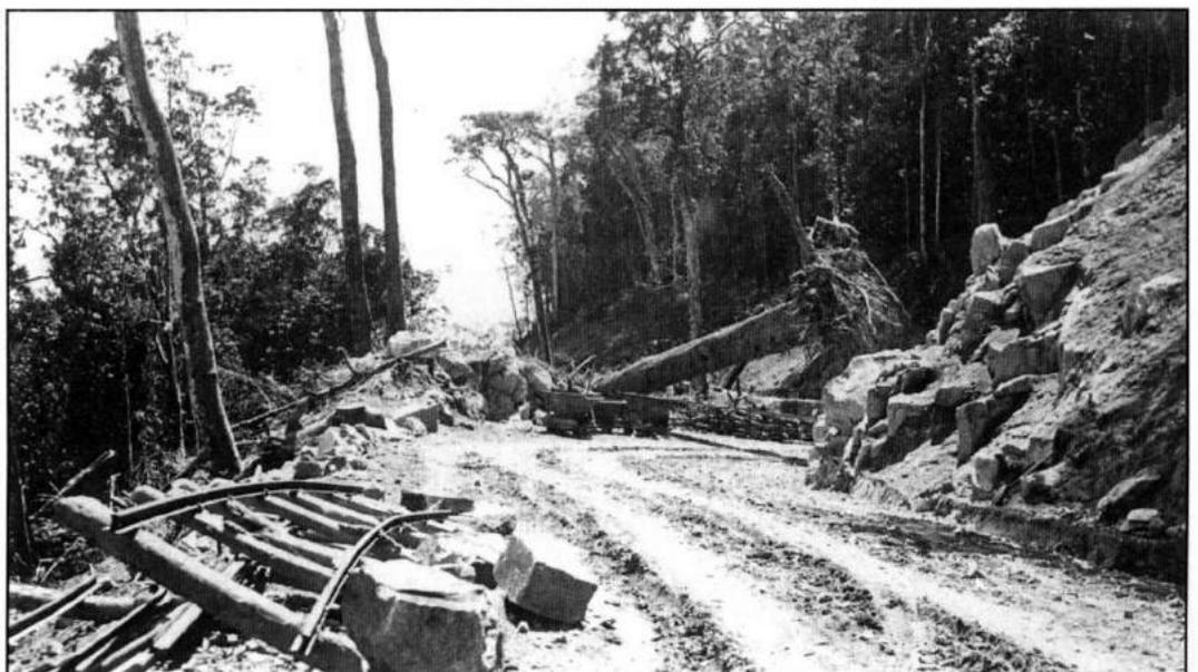
ca1933 Mt Spec Road. View of a large maple balanced on the edge of Mt Spec Road during construction. Note the use of mining technology – tramlines and trolleys.
