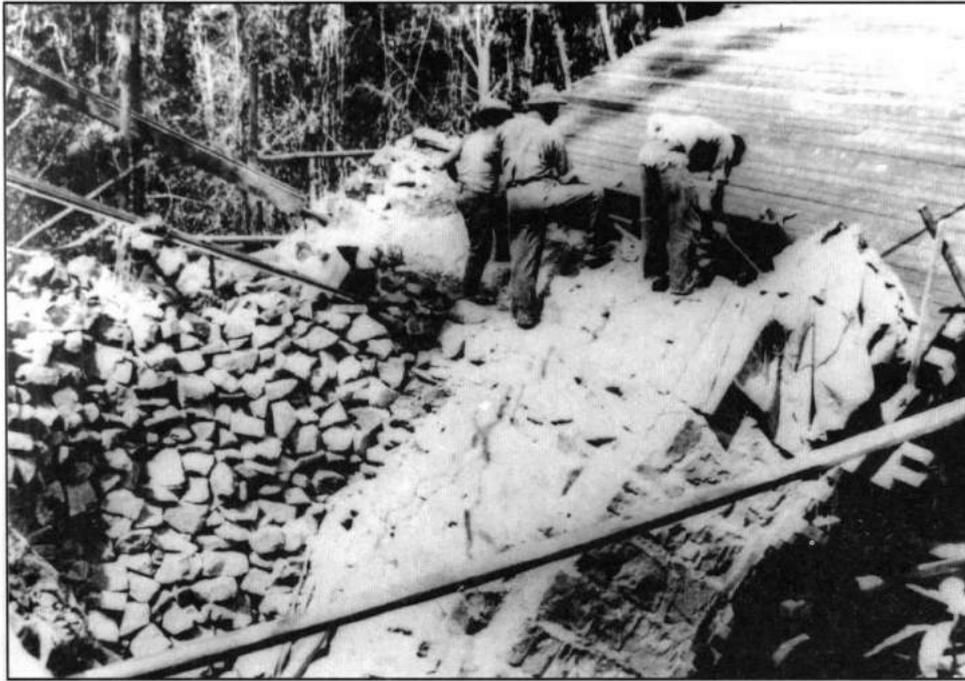
10 October 1932 Little Crystal Creek, Mt Spec Road. Abutment 'B' looking due south. Note the lagging put down on the formwork to hold the concrete when it was poured over the rock fill.
