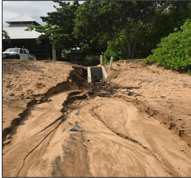
FIGURE 3-28 STORMWATER OUTFALL DISCHARGE AND EROSION DURING FEBRUARY 2018
