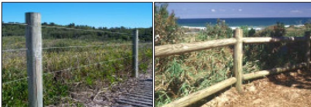
FIGURE 5-9 EXAMPLES OF PLAIN WIRE FENCING (LEFT) AND POST AND RAIL FENCING (RIGHT) (SOURCE: DECCW, 2010)
