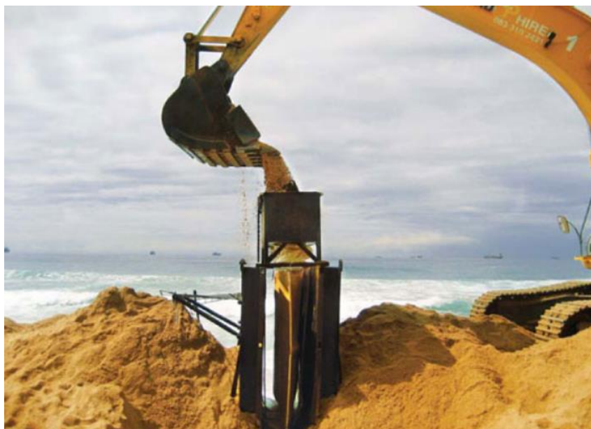
FIGURE 5-11 EXAMPLE OF DRY-FILLING A GSC WITH A FRAME (SOURCE: CORBELLA, 2012)
