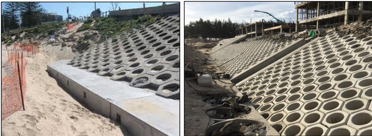
FIGURE 5-10 CONCRETE SEABEE SEAWALL - POSSIBLE TOE DETAIL (LEFT) AND SEABEE WALL DESIGNED BY WATER TECHNOLOGY (2016) (RIGHT)
