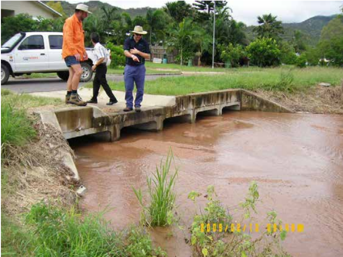
Figure 5.5.2: Sediment in the culvert under Gifford Street where Beeran Creek East discharges into the park.
