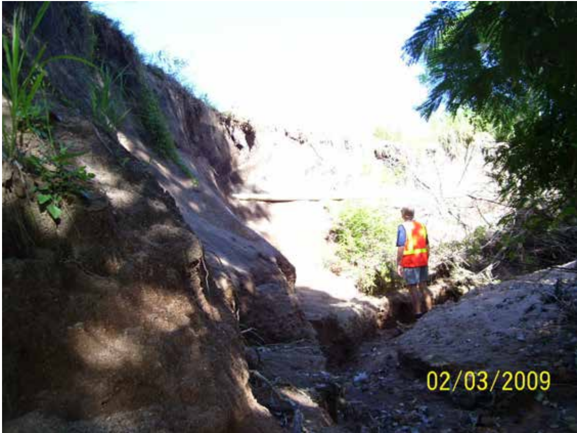
Figure 5.5.1: Beeran Creek East upstream of Gifford Street showing an exposed pipe due to extensive washout within the channel.
