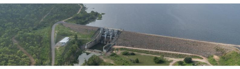
The Ross River Dam was built in the 1970's and serves two primary functions, flood attenuation and water supply.
