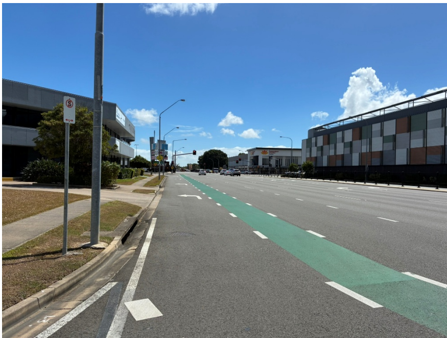
Figure 7 - Nathan Street facing North
