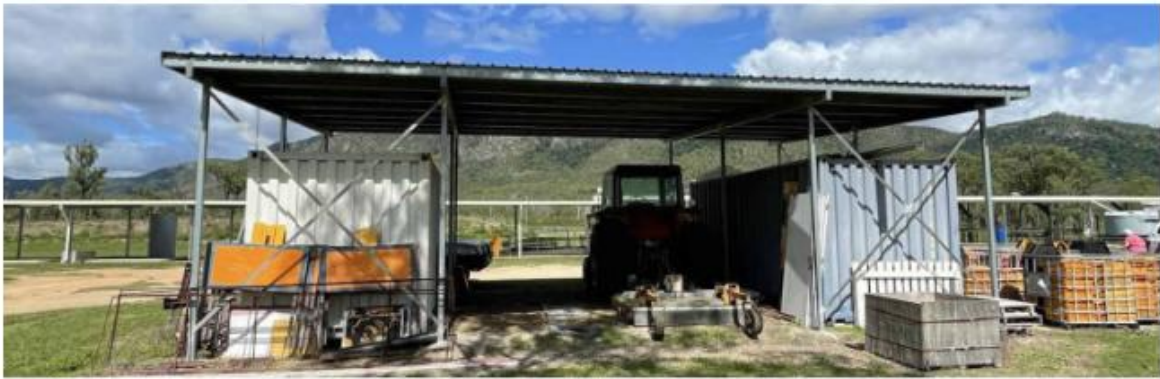
BUILDING 10 - AWNING OVER SHIPPING CONTAINERS NOT FIXED TO GROUND
