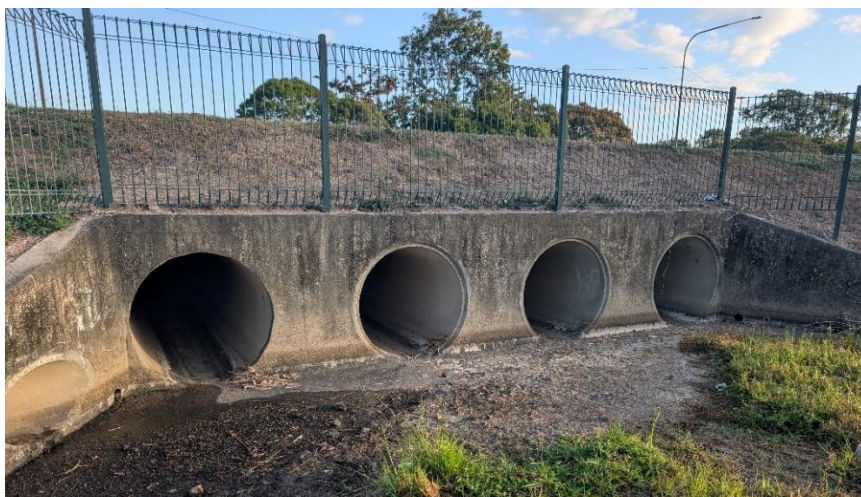
Figure 2.2 – Existing culvert under Percy Street (Site Photo)
