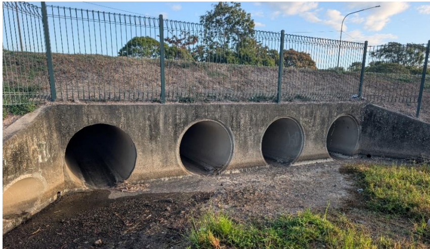
Figure 2.2 – Existing culvert under Percy Street (Site Photo)
