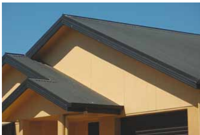
Figure 5 A dark-coloured roof absorbs and re-radiates heat (Photo: TCC).
