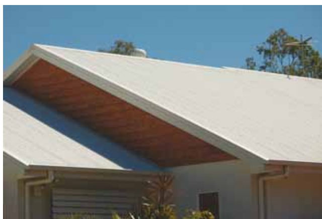
Figure 4 A light-coloured roof reflects heat and stays cooler (Photo:TCC).
