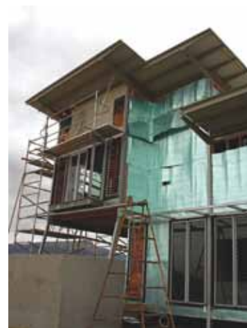
(a) During Construction
