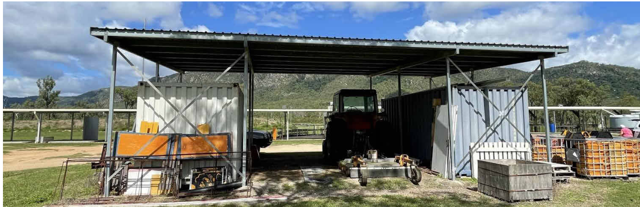
BUILDING 10 - AWNING OVER SHIPPING CONTAINERS NOT FIXED TO GROUND
