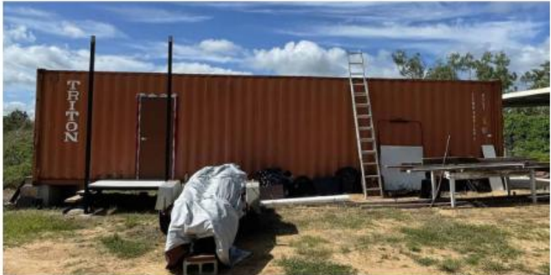
BUILDING 13 SHIPPING CONTAINER - NOT FIXED TO GROUND
