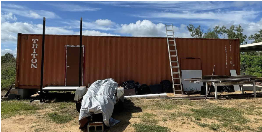
BUILDING 13 SHIPPING CONTAINER - NOT FIXED TO GROUND
