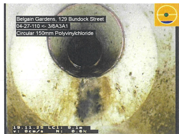
474017_46f3a490-3c7f-433f-a6f6-223ba76ddb3c_20251119_105419_480.jpg, 00:05:46, 9.10 Finish node, major connection without a maintenance structure, Nodename:, 04-27-110, grid: Roughly Finish at the fence line
