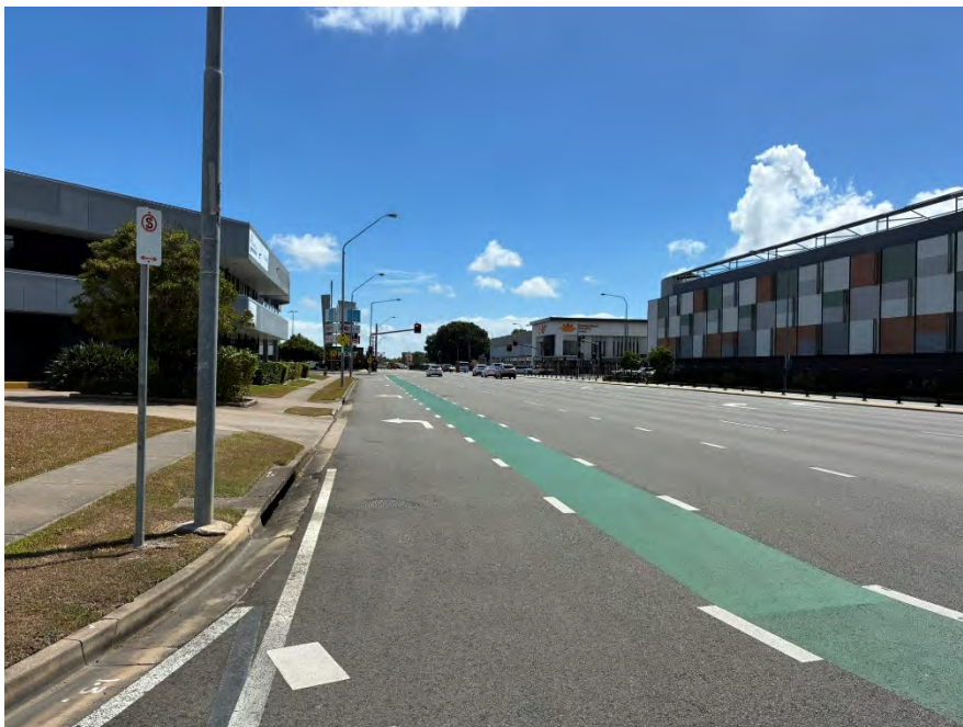
Figure 7 - Nathan Street facing North
