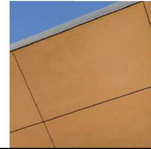
SFT-01 PRE-FINISHED FIBRE CEMENT SOFFIT
