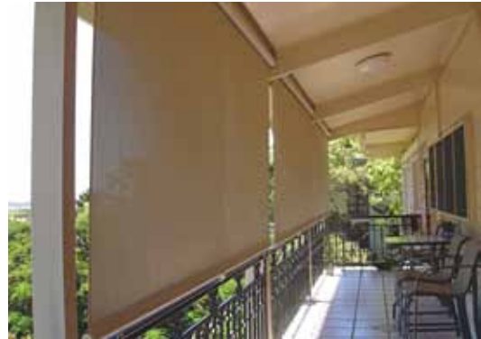
Figure 8 Adjustable blinds on the eastern side of this deck provide shade from the low-angled morning sun (Photo: ecoSAVVY).
