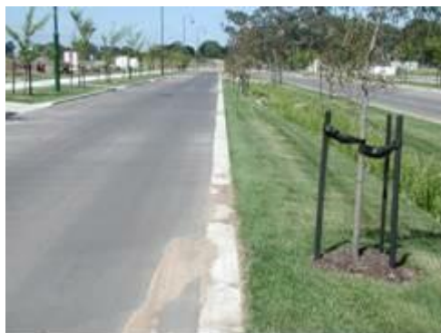
Figure SC6.4.3.9.6 Flush kerb without setdown, showing sediment accumulation on road
