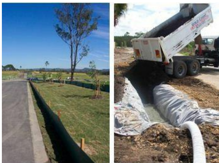
Figure SC6.4.3.9.14 Bioretention swale functional installation
