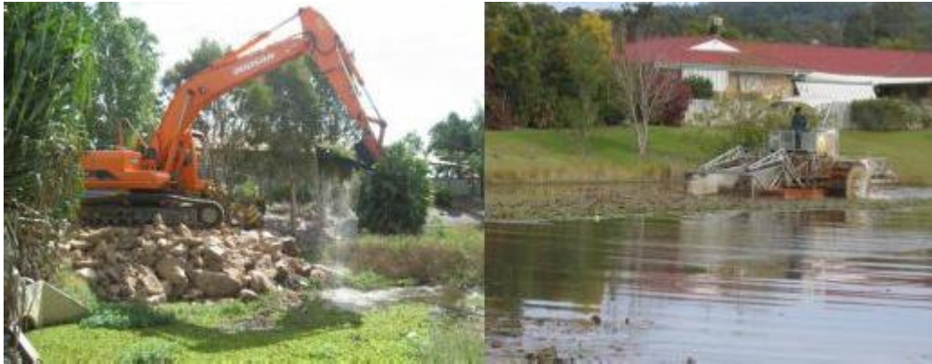
Photos: Jason Lange, and Sunshine Coast Regional Council and Ecological Engineering
