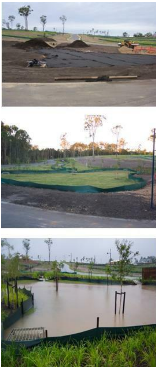
Figure SC6.4.3.9.21 Bioretention basin sediment and erosion control
