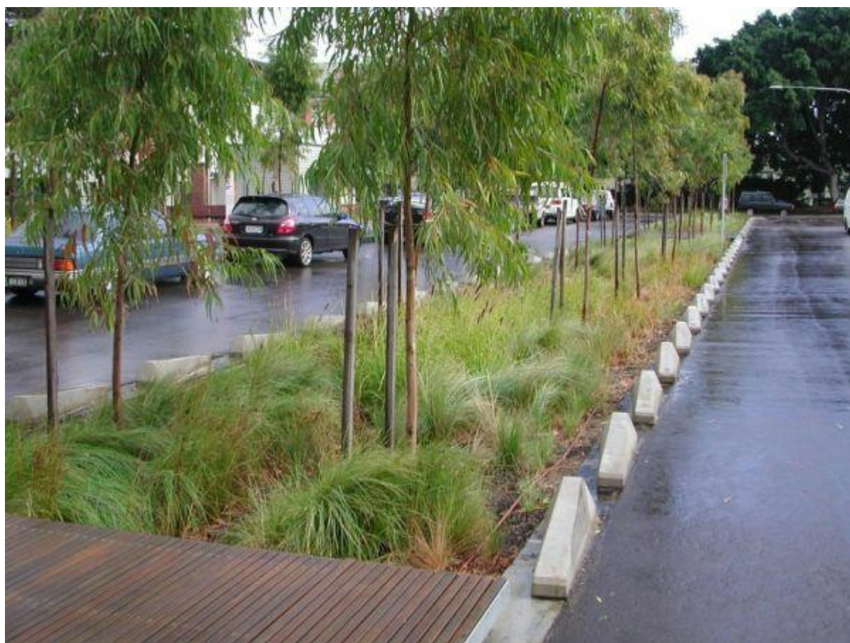
Figure SC6.4.3.9.9 Median strip bioretention applications
