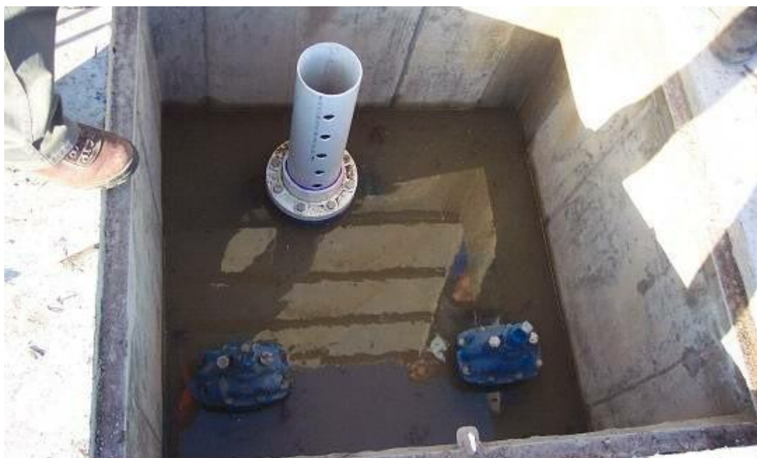
Figure SC6.4.3.9.36 Macrophyte zone outlet arrangement
