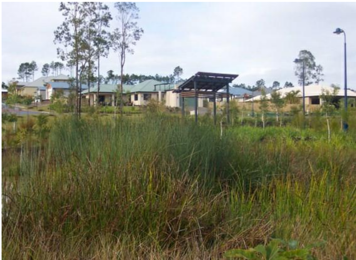
Figure SC6.4.3.9.46 Constructed wetland operational establishment
