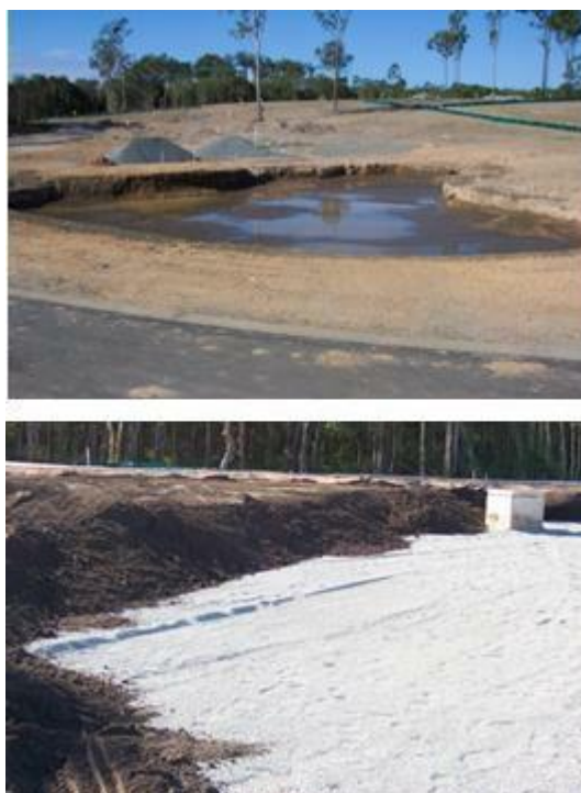
Figure SC6.4.3.9.20 Bioretention basin functional installation
