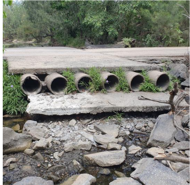
Figure 4- Culvert causeway
