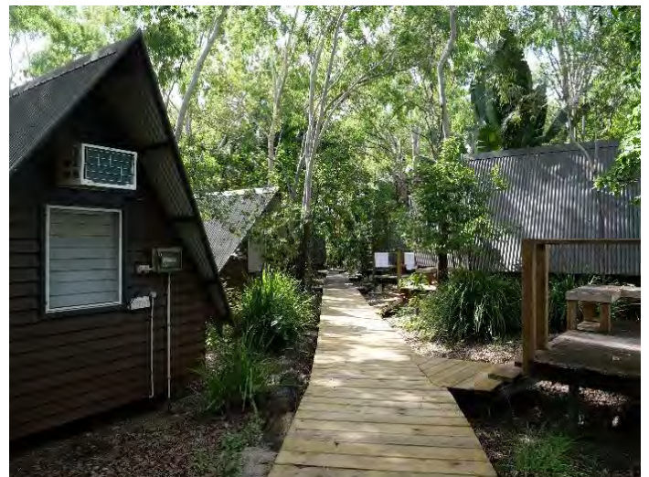
FIGURE 11 VIEW OF REAR OF AN EXISTING ACCOMOTATION WITH DECKING PATHWAY ON SUBJECT SITE.
