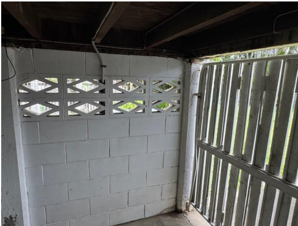
Figure 4 Un-reinforced 100mm screen blocks
