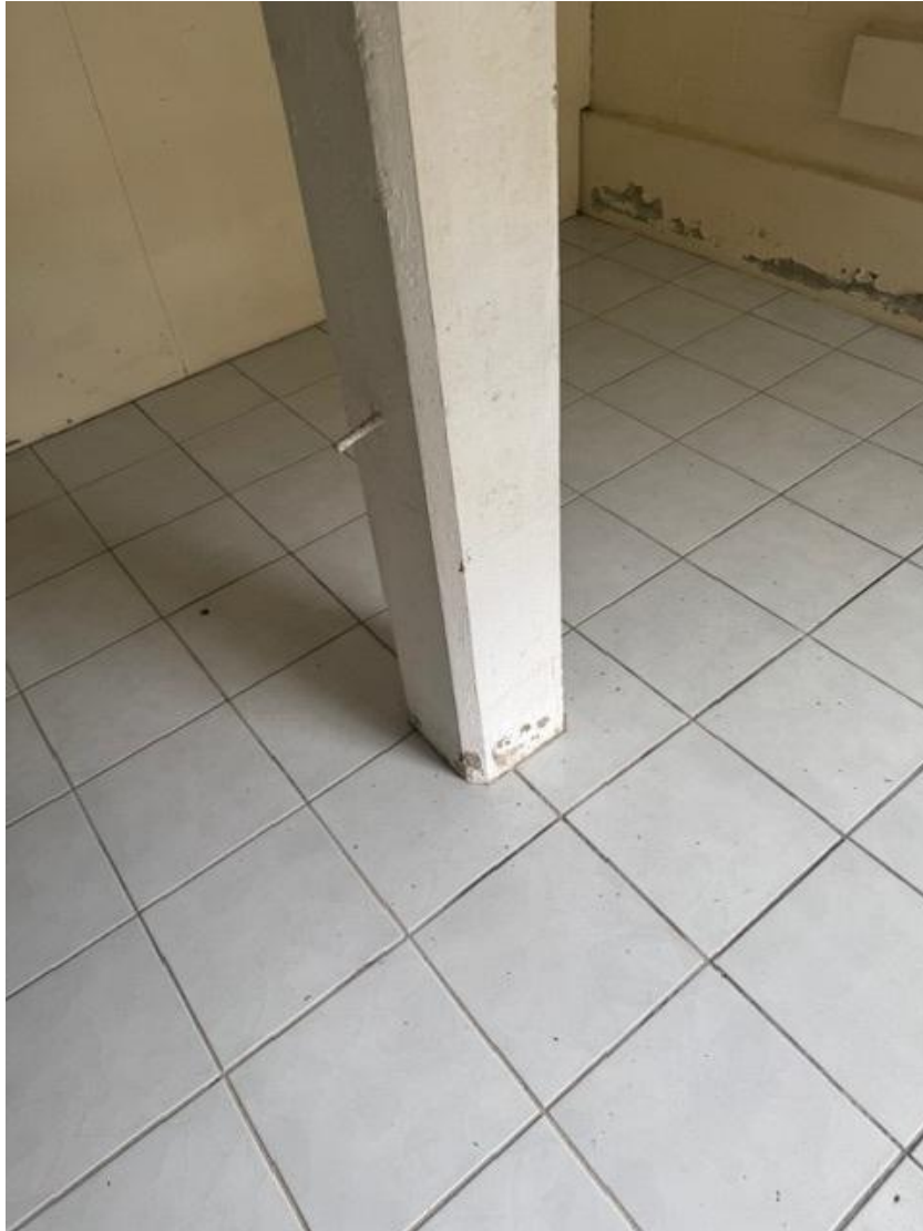
Figure 10 Missing Bracing & Bolt Protrusion
