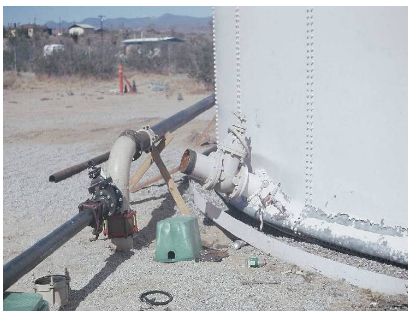
Figure 3.15: 'Elephant's foot' damage to a large metal water tank caused by earthquake shaking (American Public Works Association photo)
