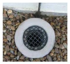
The ORG is fitted at a depth lower than the floors in your house that have waste outlets, such as bathrooms, toilets and the laundry. If a sewerage blockage occurs, the ORG grate should pop off to release the pressure and direct sewage away from the home.
