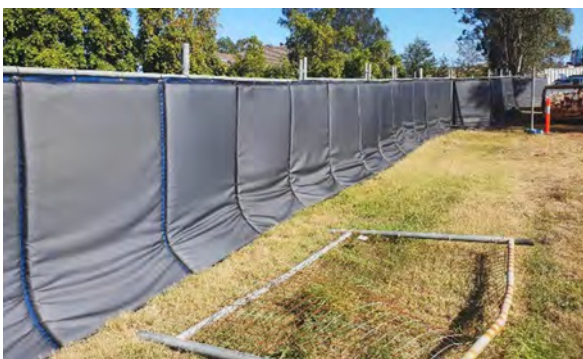
Figure 23 Temporary noise fencing - Sound Block Acoustic Barrier (source: https://fortressfencing.com.au/sound-block-acoustic-barrier-noise-barrier ).
